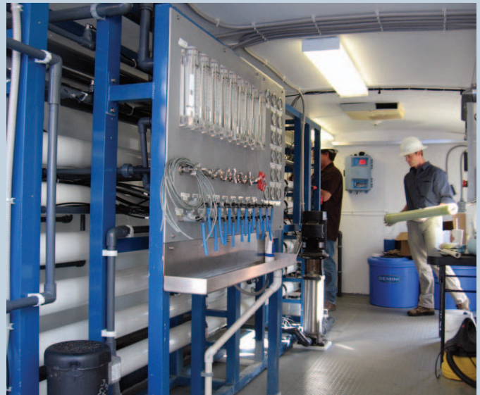
Membrane filters installation
