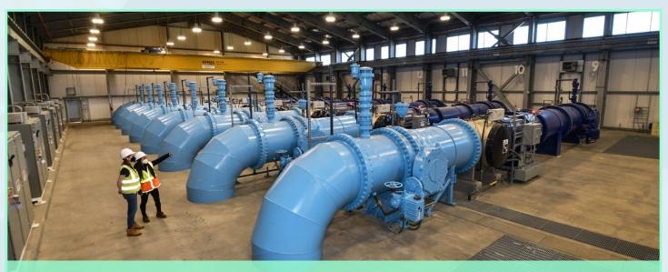
LADWP engineers inspect some of the 15 UV reactors at the LARUVDP designed to provide high-quality drinking water.
