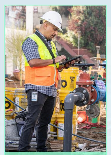
An LADWP Water Service Representative inspects a backflow installation at a construction site at USC Medical Center. The use of a new iPad loaded with the new CCCU Dispatch Application software, ensures timely and efficient inspections that safeguard water quality in the City's distribution system.
