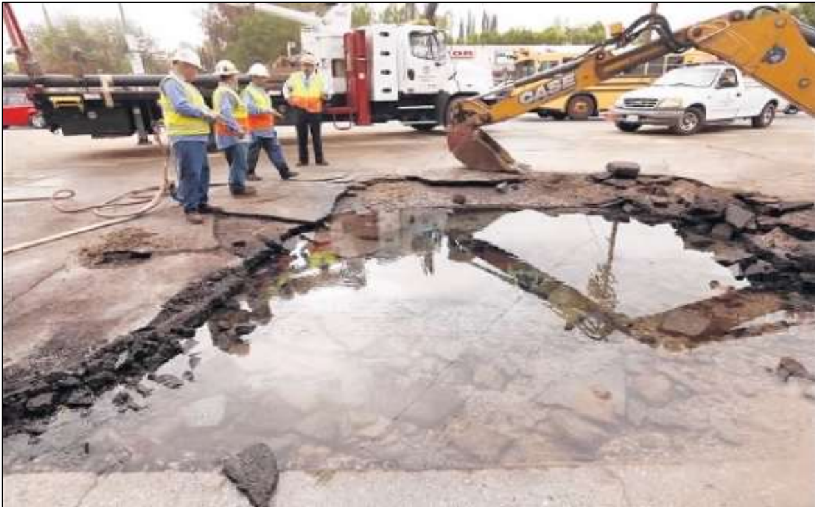
Plate 2: Rupture repair at Tampa Avenue and Topham Street, 2017 ( Los Angeles Times 2017)
