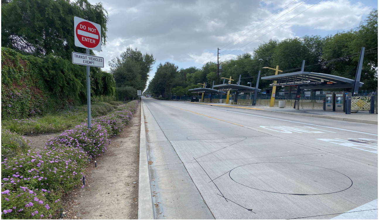
Photo 2: South-facing view of Orange Line Busway bike path along Victory Boulevard.
