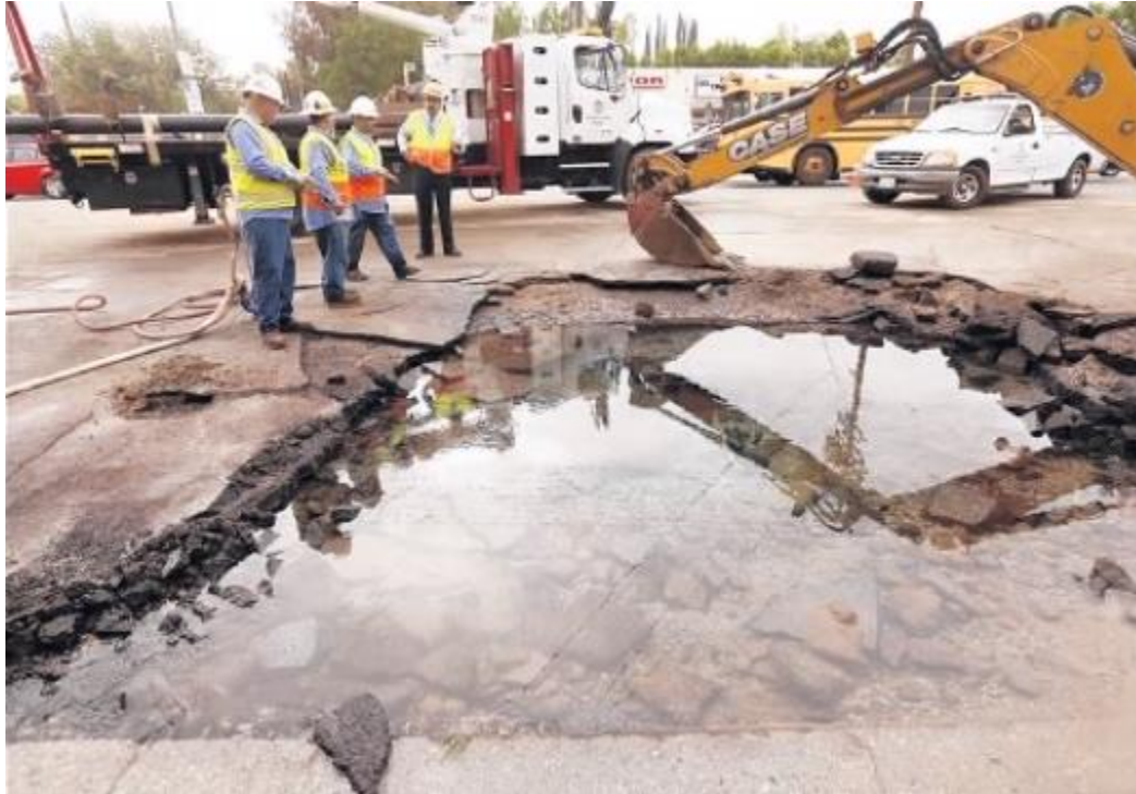
Plate 3: Rupture repair at Tampa Avenue and Topham Street, 2017 ( Los Angeles Times 2017)
