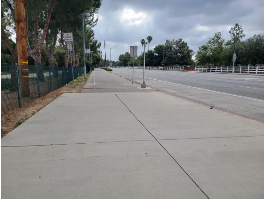
Photograph 3. Overview of an underground section at Mason Avenue and Victory Boulevard, view to east, April 28, 2022
