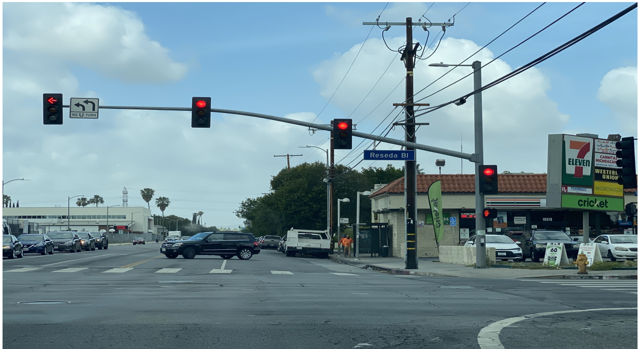
Photo 7: North-facing view along Oxnard Street at intersection with Reseda Boulevard.
