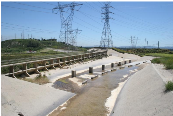
Mid Portion of Channel Convergence, Exp. 1934, View to Southeast
