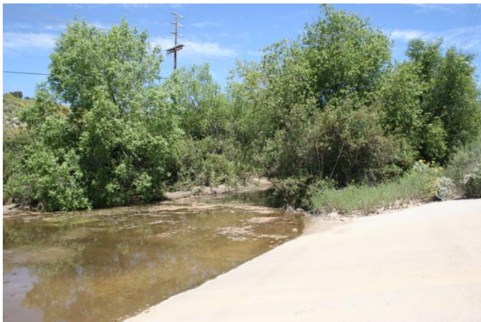
Northern Portion of BCEC Near Intersection of Balboa Boulevard and San Fernando Road, Exp. 1906, View to North.
