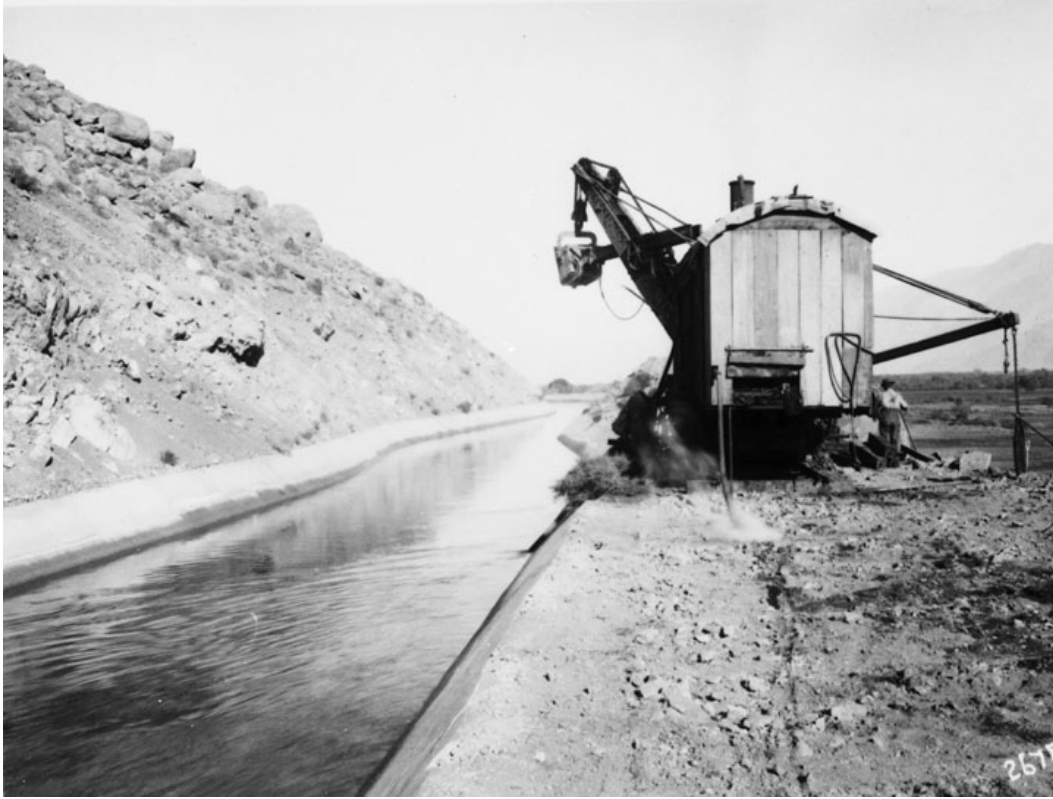
Plate 3. Steam Shoveling Along the Los Angeles Aqueduct N.D. (LAPL, LADWP Photo Collection)
