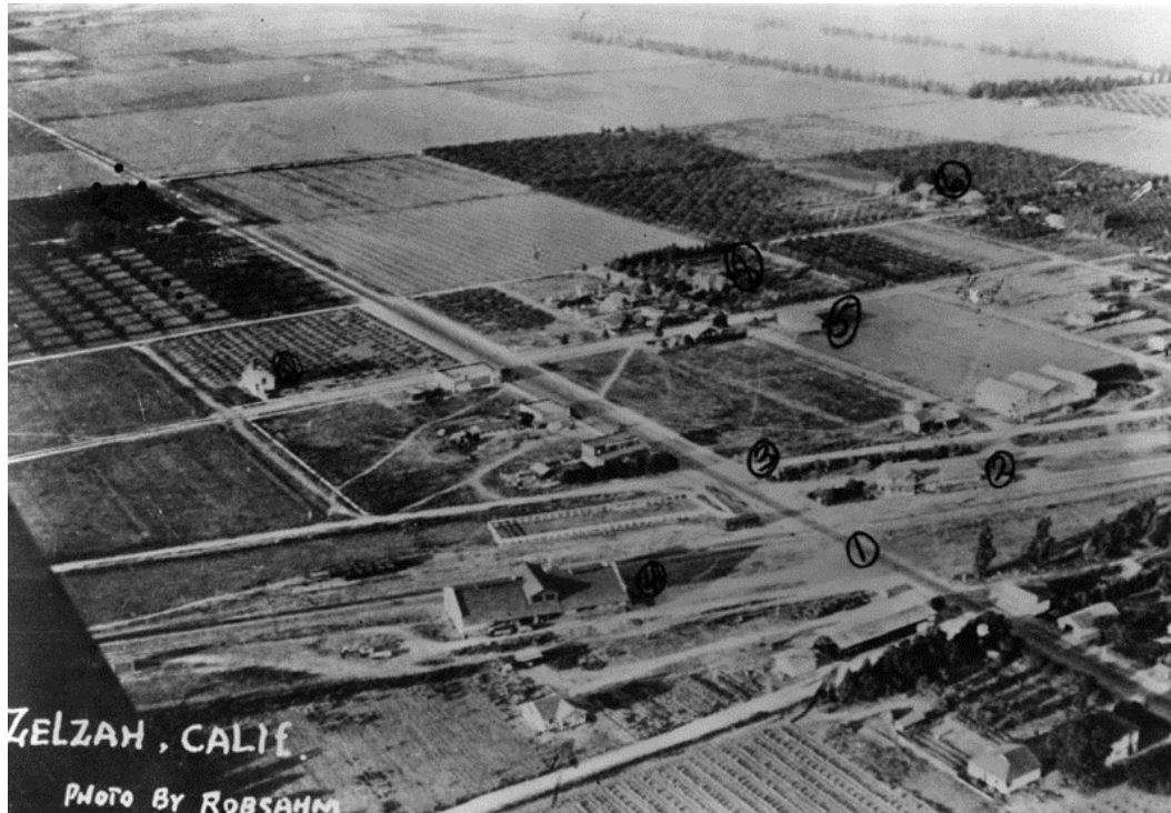
Plate 3. Aerial View of Zelzah, View Northeast. Reseda Boulevard Marked 1, Southern Pacific Depot Marked 2, Parthenia Street Marked 3 (LAPL 1918).
