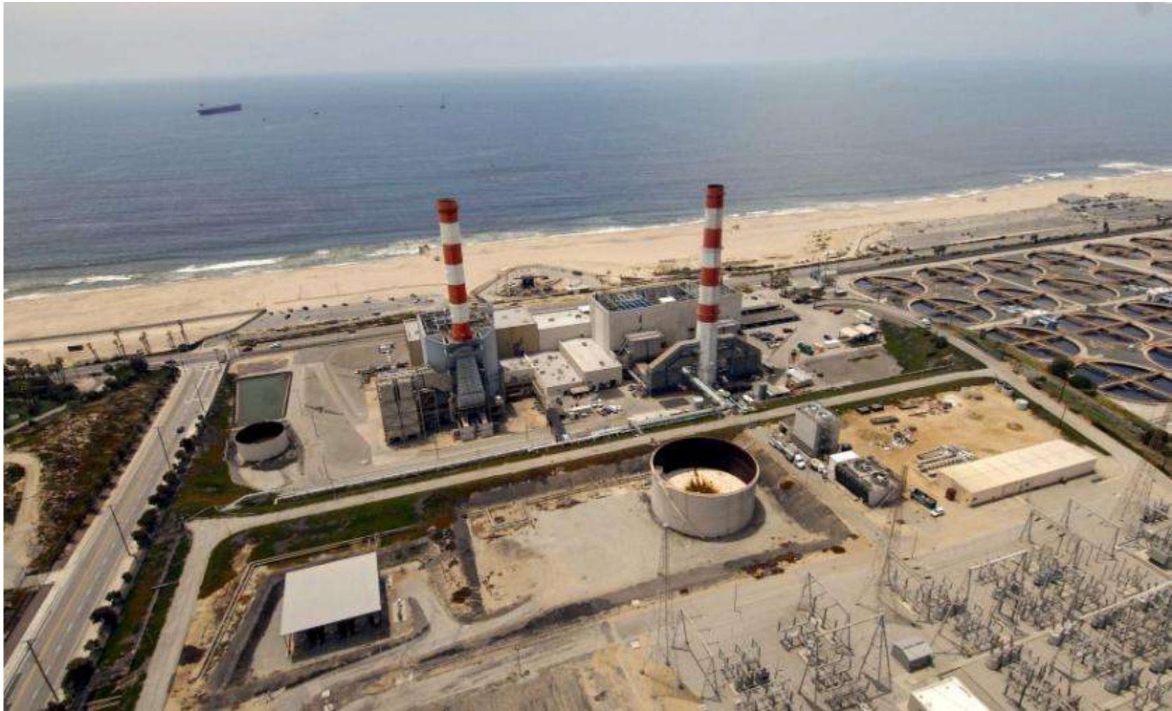
FIGURE 3.3-3. SITE FACILITIES – FROM LEFT, UNIT 3 WITH STACK, AND UNITS 1 AND 2 WITH SHARED STACK
