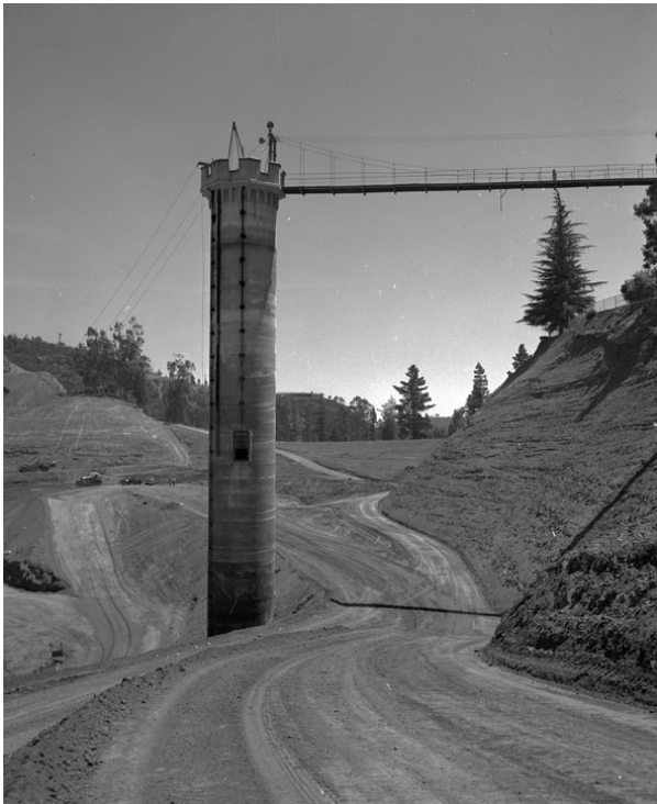
Plate 3. Outlet Tower and Foot Bridge, circa. 1953 (LAPL DWP Photo Collection 1004919)
