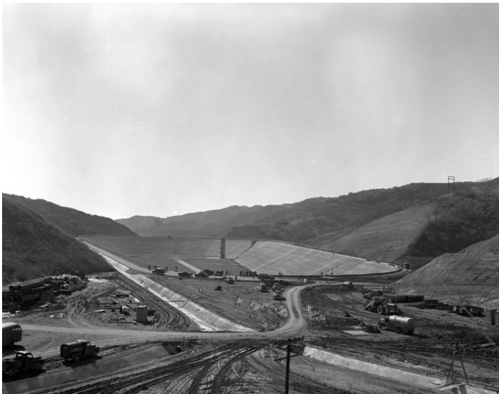
Plate 2. Construction of Upper Stone Canyon Reservoir, circa 1953 (LAPL DWP Photo Collection 1004923)
