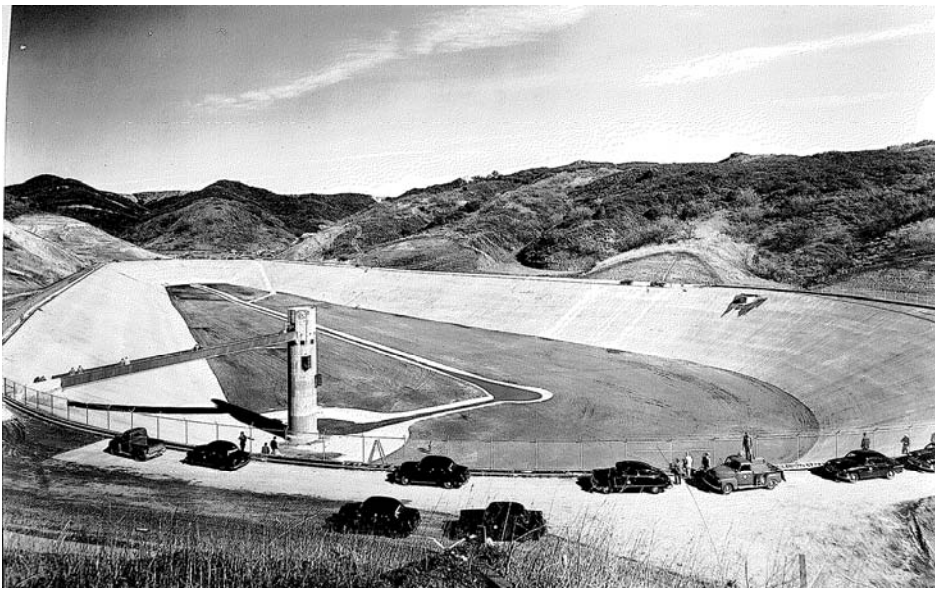
Plate 4. First Water Entering Upper Stone Canyon Reservoir (January 27, 1954) (Hayward 1956)
