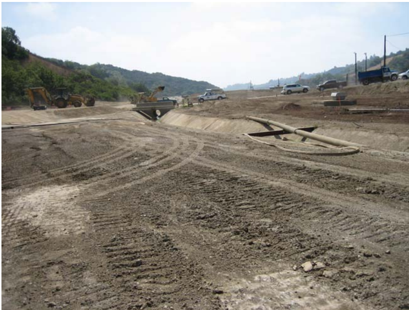
Plate 6. Graded Portion of Project Area North Reservoir, View to South.
