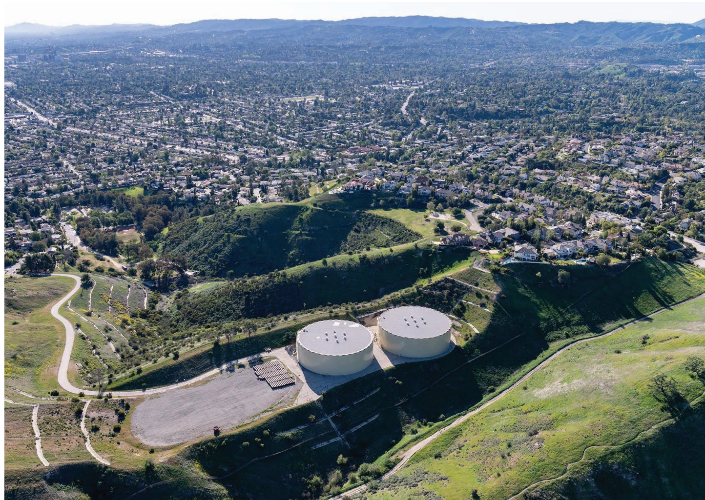
The Kittridge Water Tanks located in West Hills can each hold 10-million gallons of water.
