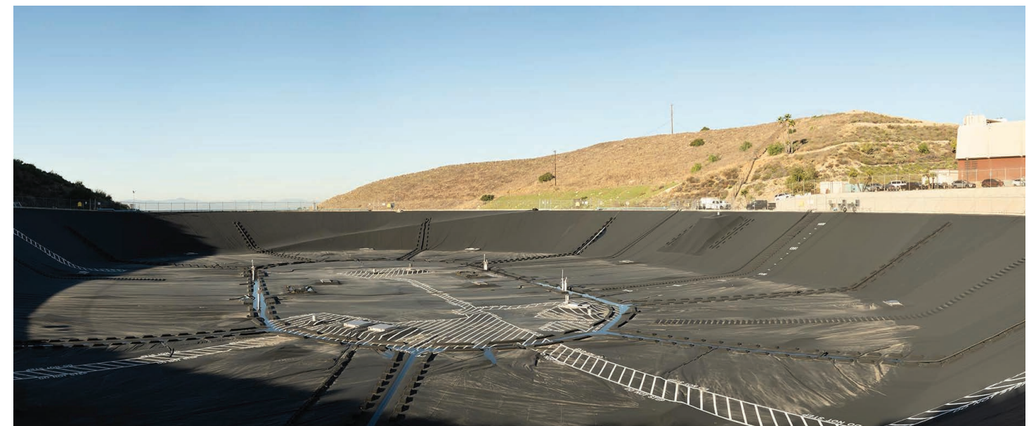
The floating cover on the Green Verdugo Reservoir adjusts as needed to the changing water levels.
