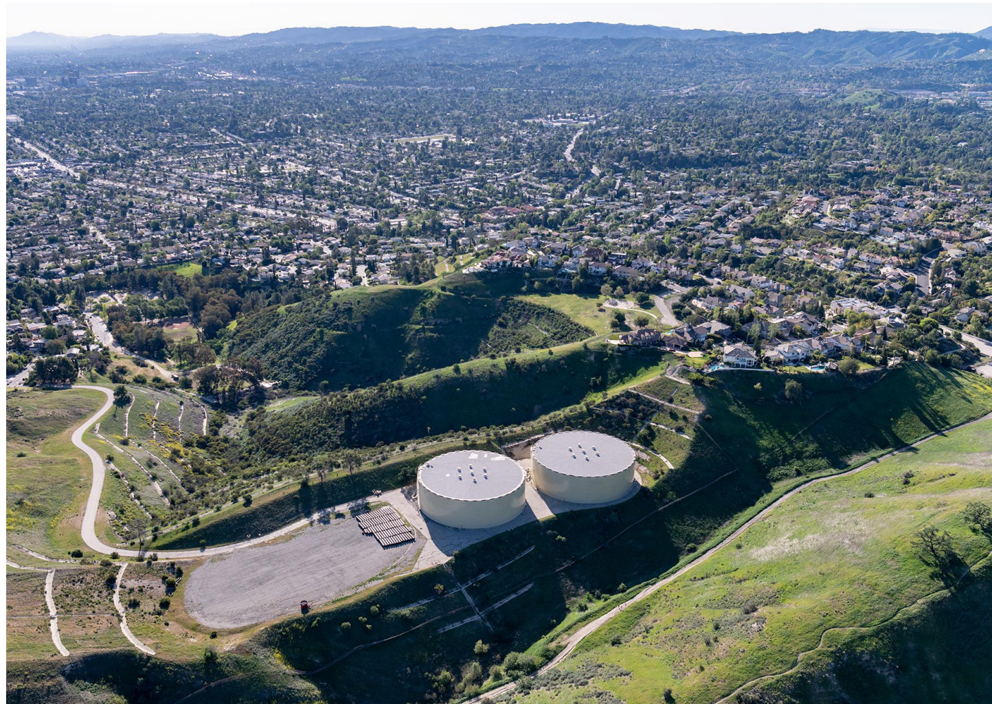
The Kittridge Water Tanks located in West Hills can each hold 10-million gallons of water.
