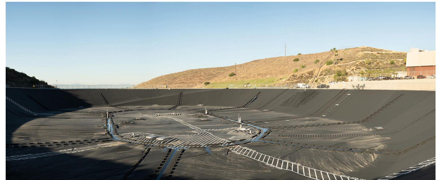
The floating cover on the Green Verdugo Reservoir adjusts as needed to the changing water levels.
