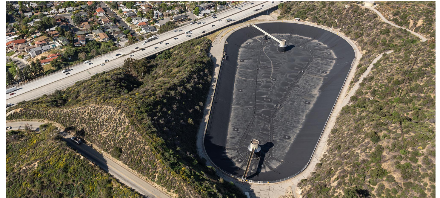
The floating cover on the Eagle Rock Reservoir provides added protection to L.A.'s drinking water.
