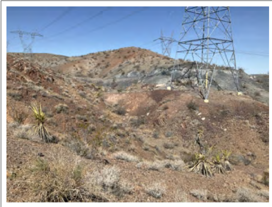
View of Drainage 06-CR-015. View of typical drainage conditions in hilly portion of survey area. Photo taken May 4, 2022.
