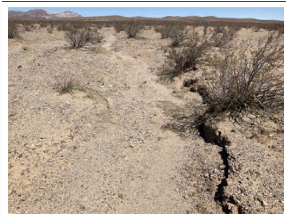
View of Drainage 08-MI-112. Typical sandy wash. The scour line leaving a near-vertical stream bank is common in many drainage features. Photo taken May 11, 2022.
