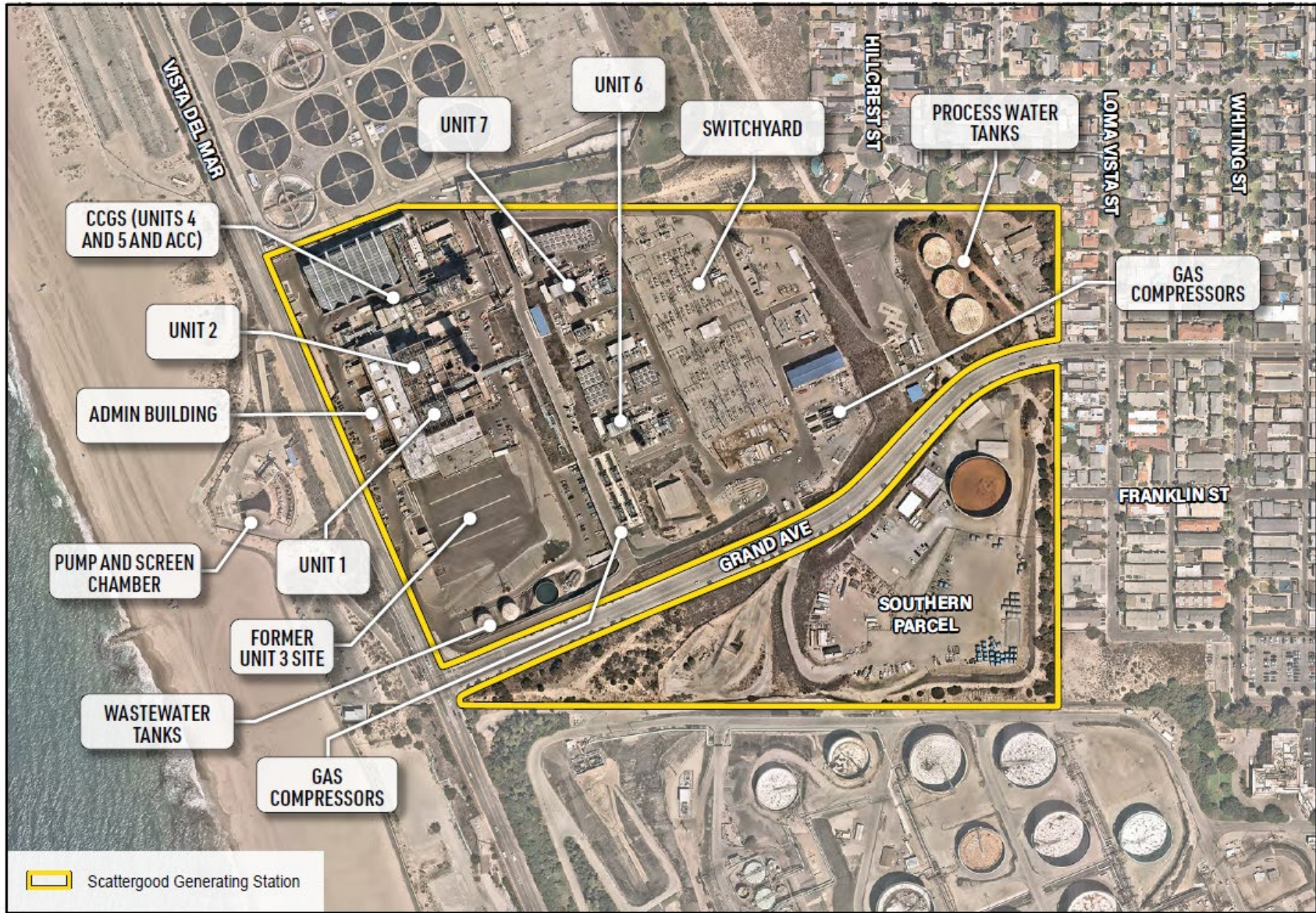
SCATTERGOOD GENERATING STATION UNITS 1 AND 2 GREEN HYDROGEN-READY MODERNIZATION PROJECT
