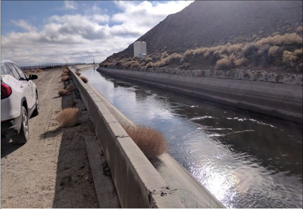
Photograph 17 – Los Angeles Aqueduct at Alabama Gates.
