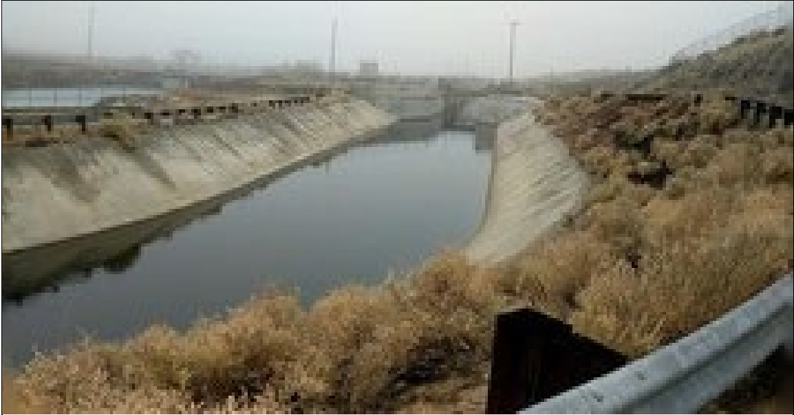
Photograph 5 – Merrit Cut and segment of aqueduct.
