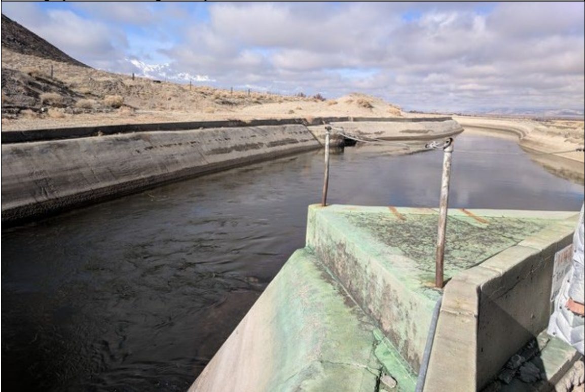
Photograph 18 – Los Angeles Aqueduct at Alabama Gates showing platform where copper sulfate application occurs.
