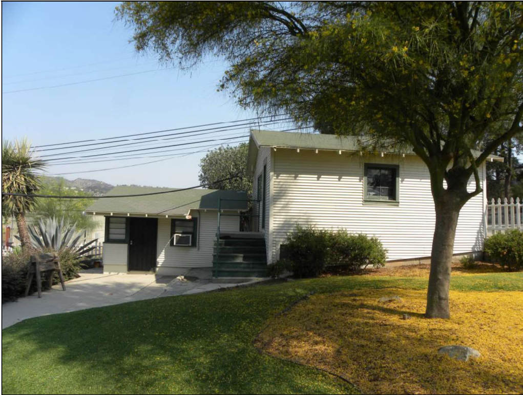
Photograph 13. Shed (left) and Garage (right), camera facing north, August 9, 2018
