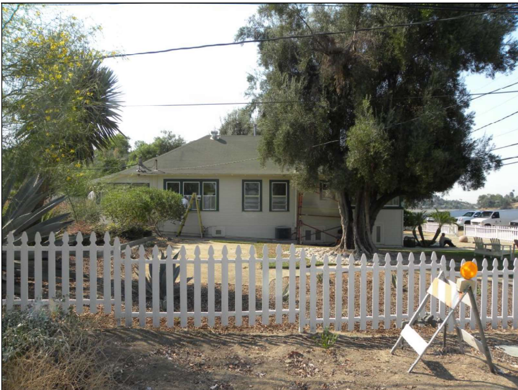
Photograph 10. New Landscaping near Caretaker's House, camera facing south, August 9, 2018
