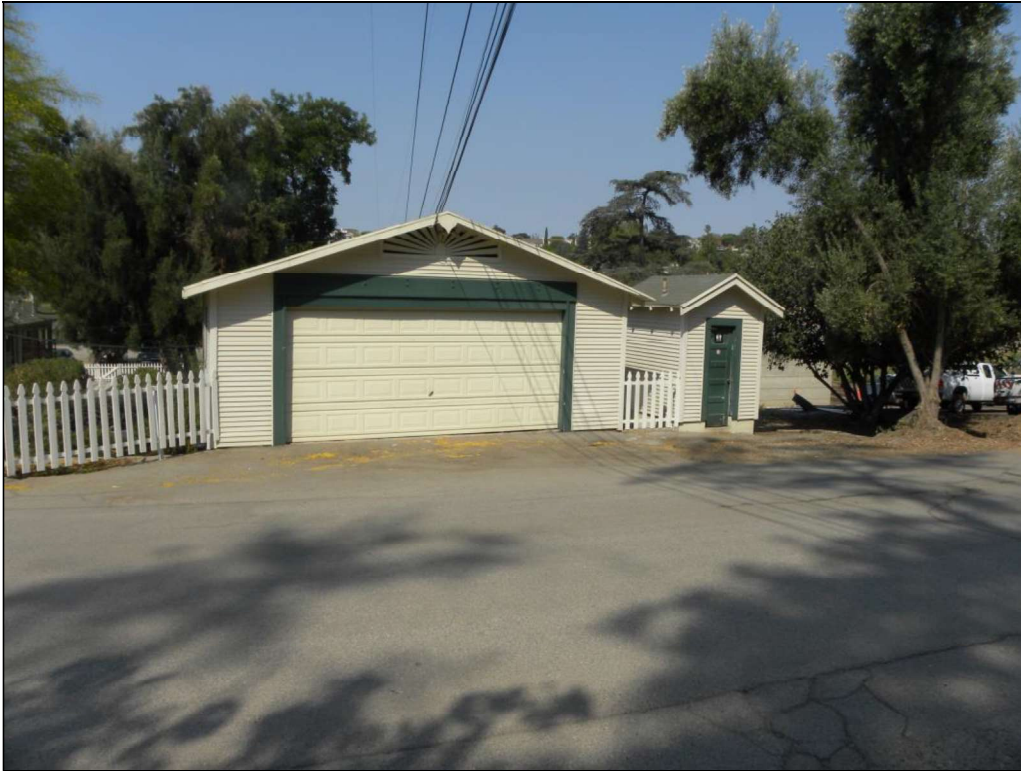
Photograph 11. Garage, camera facing west, August 9, 2018
