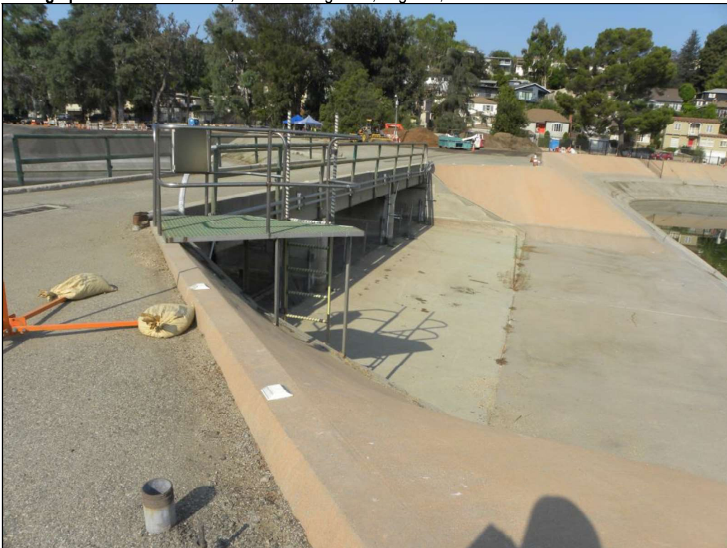
Photograph 6. Ivanhoe Dam, camera facing west, August 9, 2018
