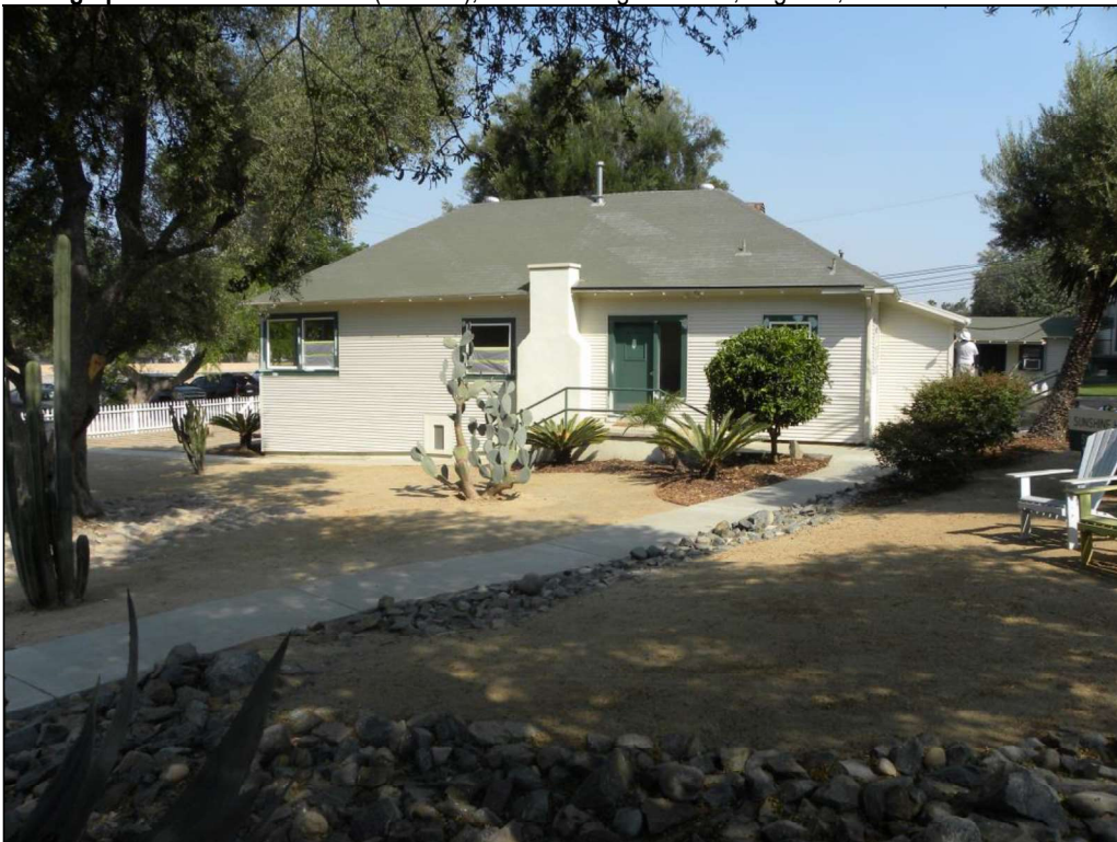
Photograph 8. Caretaker's House, camera facing north, August 9, 2018
