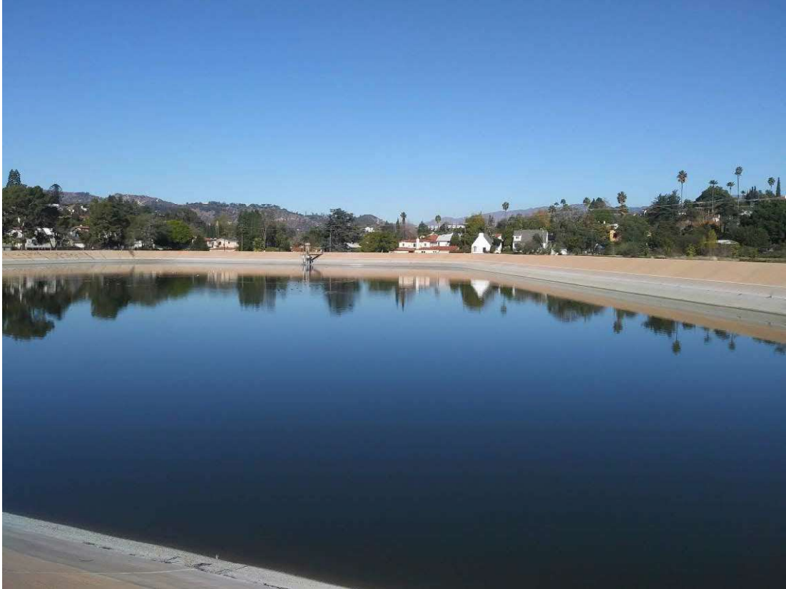
Photo 5. North-facing view across Ivanhoe Reservoir.
