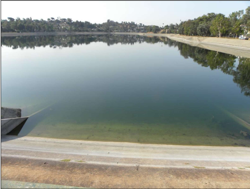
Photograph 3. Silver Lake Dam, camera facing south, August 9, 2018
