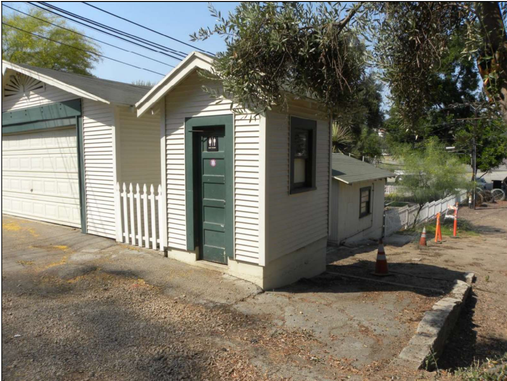
Photograph 12. Bathroom Building, note shed located behind bathroom building, camera facing southwest, August 9, 2018
