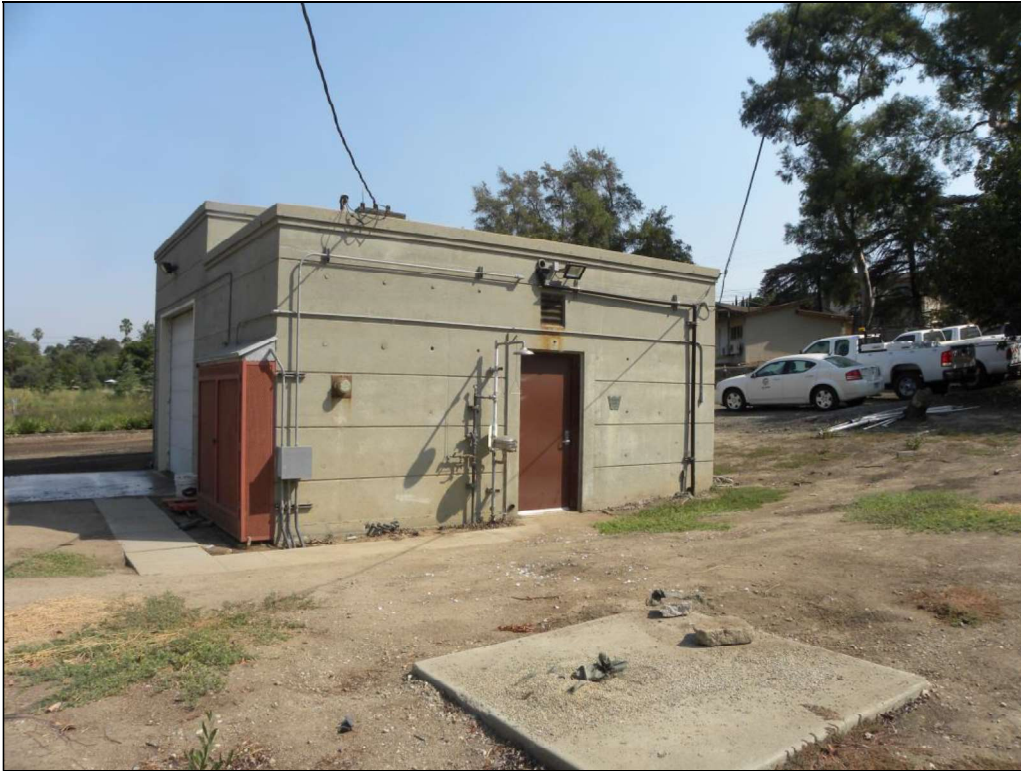
Photograph 7. Chlorination Station (Ivanhoe), camera facing northeast, August 9, 2018
