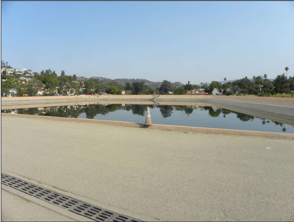
Photograph 5. Ivanhoe Reservoir, camera facing north, August 9, 2018
