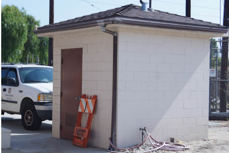
Plate 14: 99th Street Wells Pumping Station Building 3, View Facing Northeast.
