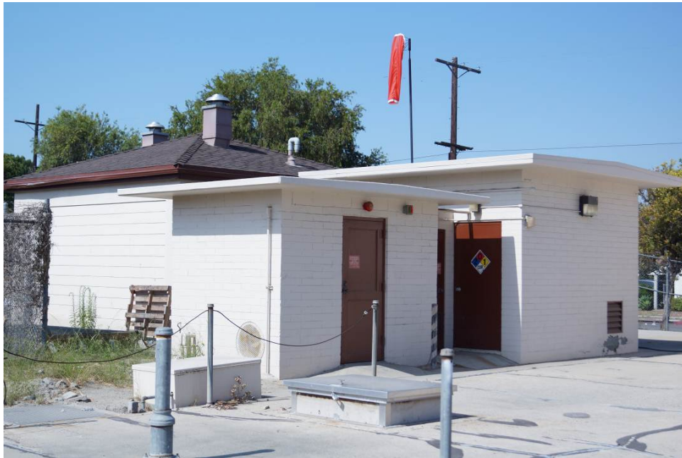
Plate 15: 99th Street Wells Pumping Station Building 4, View Facing Northwest.
