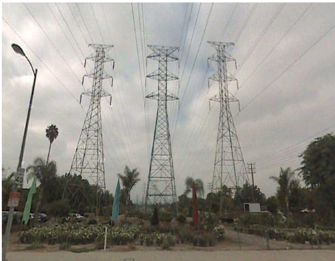
Fig. 4-22: Location for Rinaldi-Northridge, twr 248
