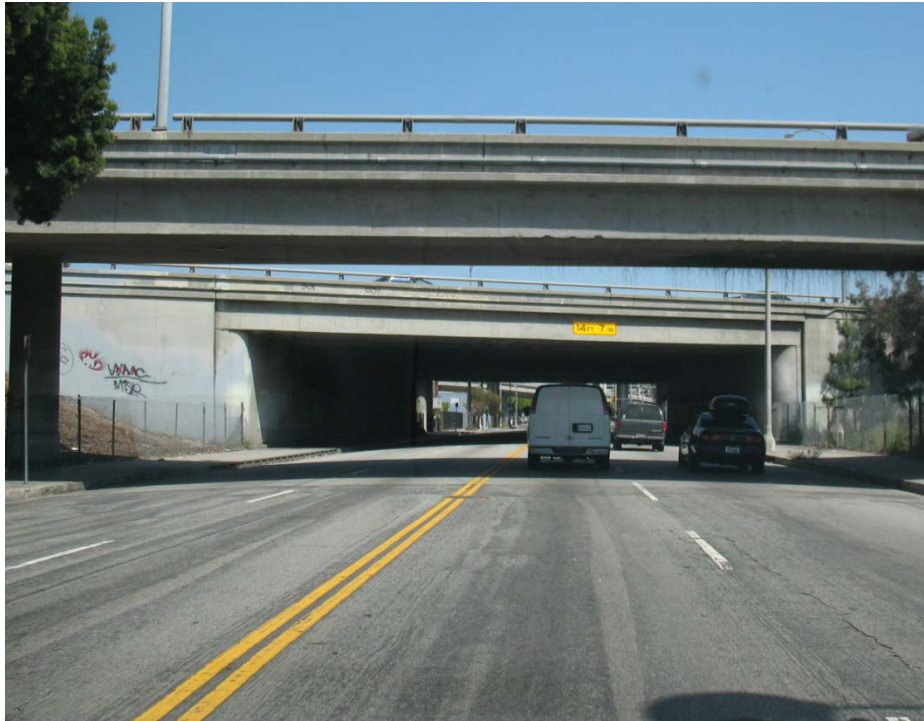
Photo 13. Photo depicting bridges and overpasses present along the Phase II proposed pipeline.
