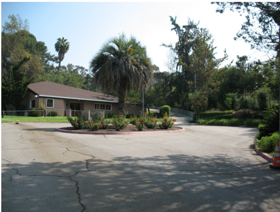
Photo 4. Photo of proposed potable water pipeline route and surrounding vegetation between Elysian Park Drive and hiking trails west of Park Drive. Photo facing north.
