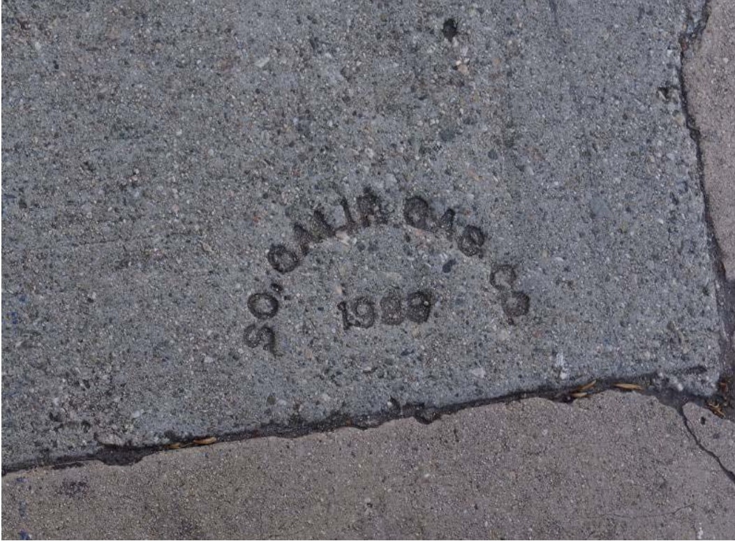
Figure 89. Sidewalk along Northbound Broadway, “SO. CALIF. GAS CO. 1929,” View South
