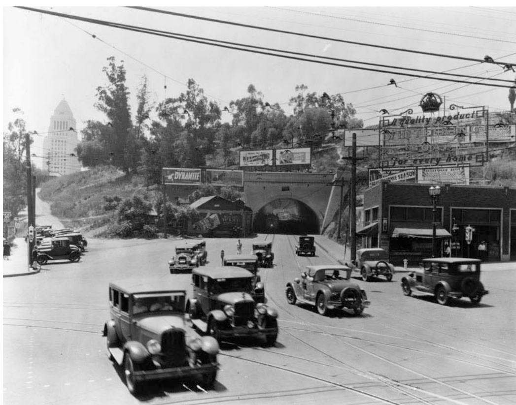
Figure 58. North Broadway and Sunset, Showing Broadway Tunnel, 1929 (Los Angeles Public Library)
