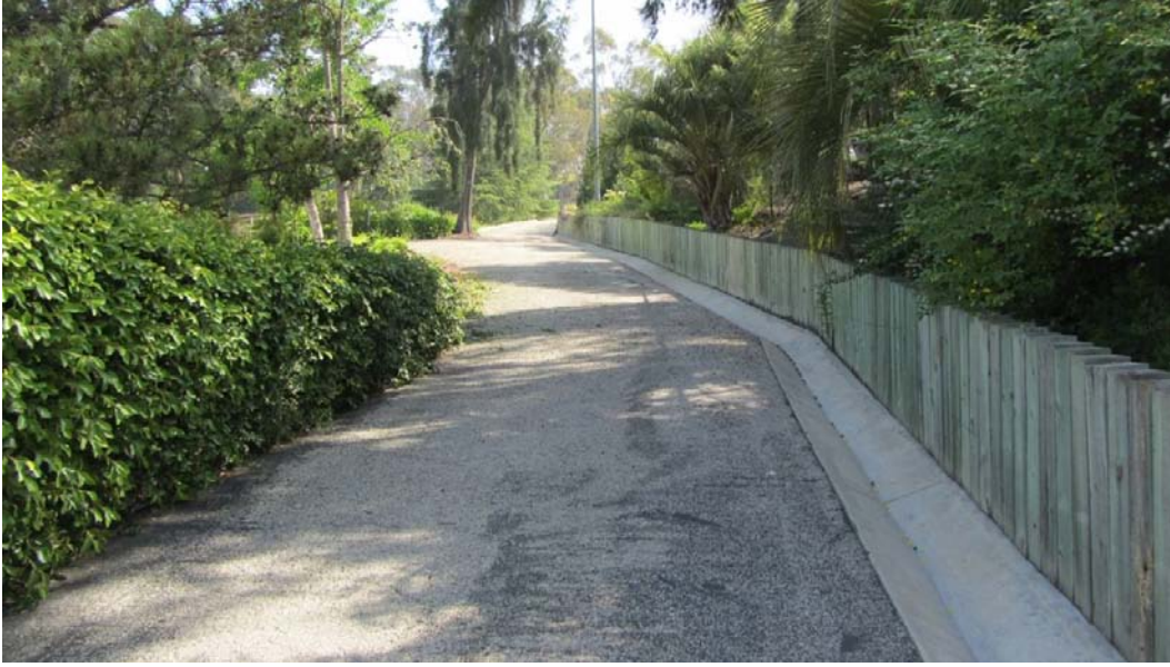
Figure 51. Utility Road Adjacent to Japanese Gardens, View Northeast
