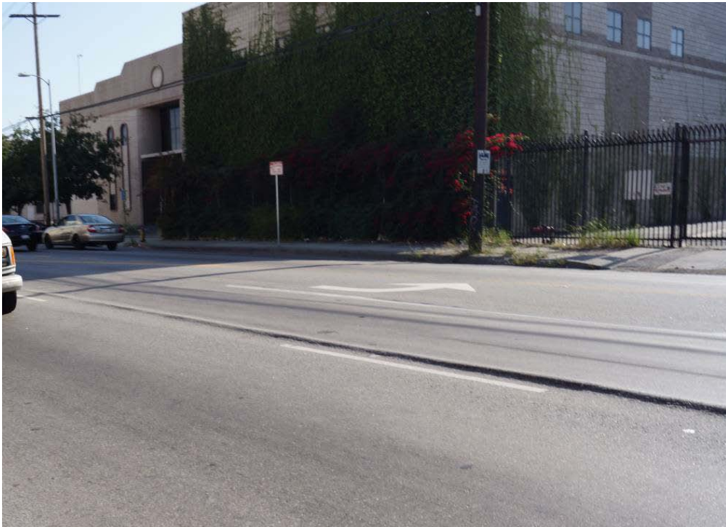
Figure 76. CA-LAN-2786, Santa Fe Avenue Railroad Tracks, View Southwest
