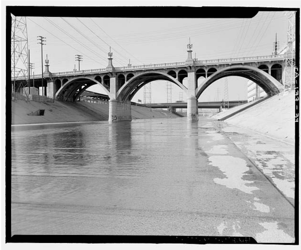
Figure 80. Olympic Boulevard Bridge/Ninth Street Viaduct, HAER Photo (Logan 1996; Library of Congress)
