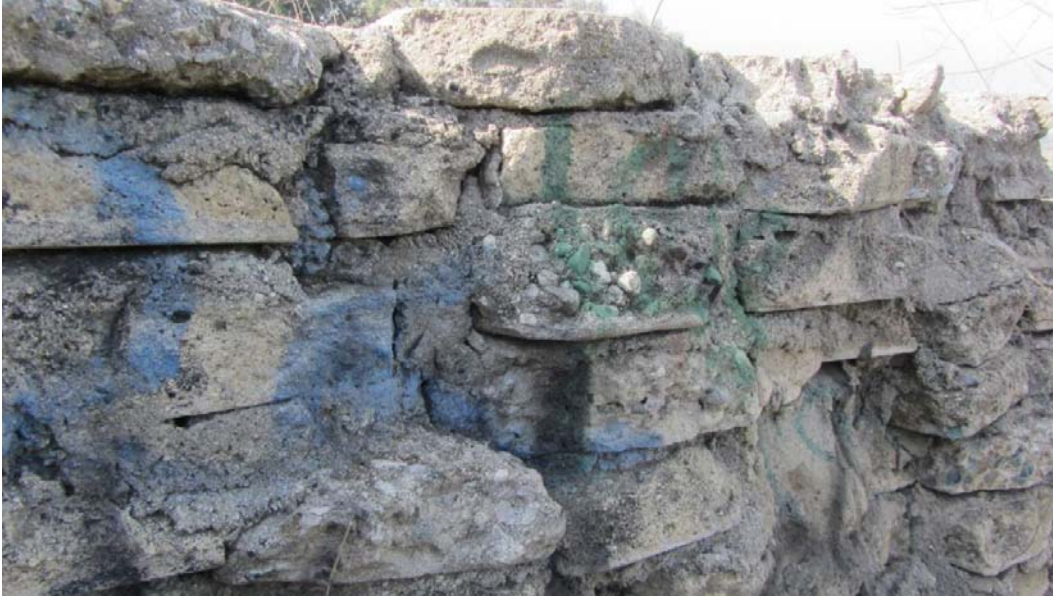
Figure 46. Close-up of Concrete Wall North Façade
