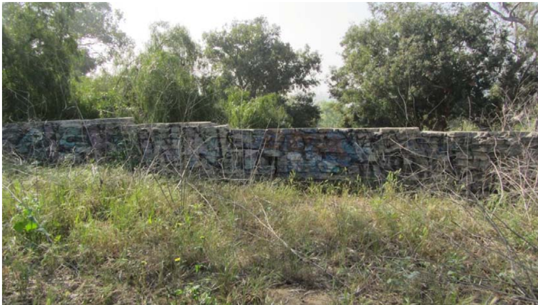
Figure 45. North Façade of Concrete Wall, View Southeast
