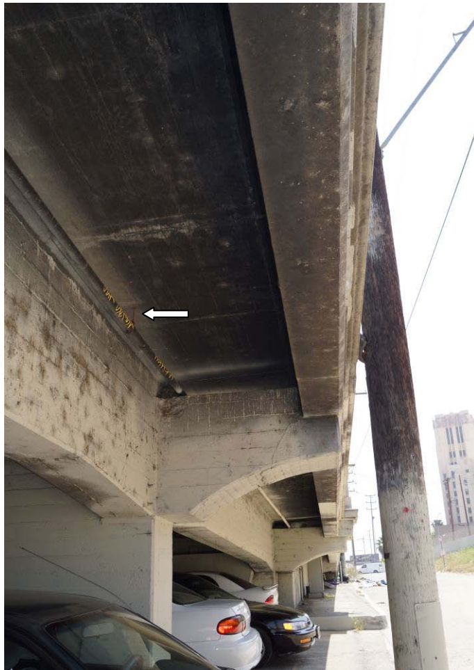
Figure 81. Olympic Boulevard Bridge, Existing Pipes, View East
