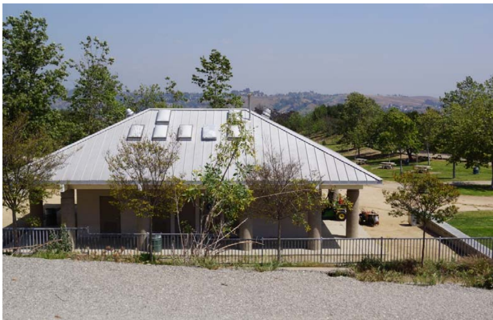
Figure 54. Public Restroom Facilities, View East
