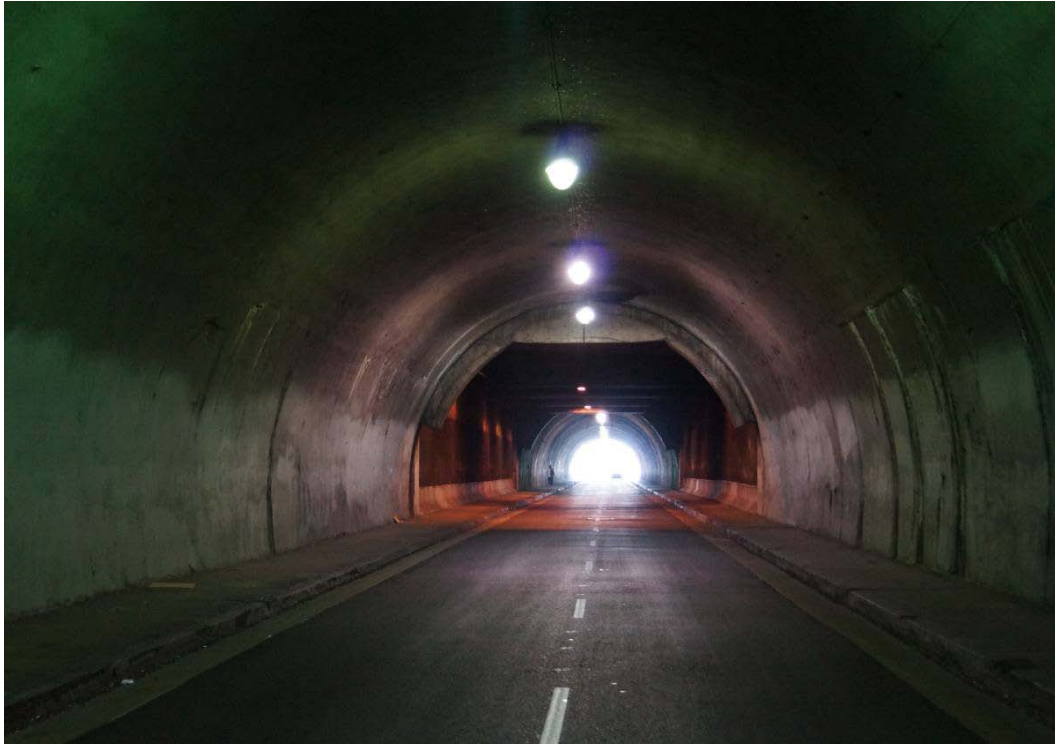
Figure 72. Third Street Tunnel, Interior, View Northwest
