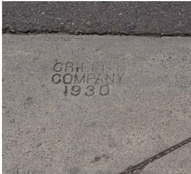
Figure 86. ELY2-H-002, Olympic Boulevard, "GRIFFITH COMPANY 1930," View South
