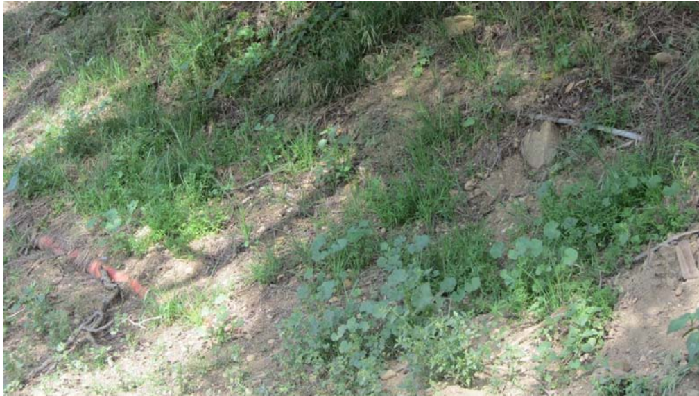
Figure 53. Exposed Water Pipes Adjacent to Fire Road, View North
