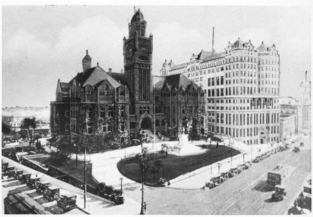
Figure 22. Los Angeles County Courthouse and Hall of Records, Broadway and Temple, 1926 (USC Digital Library)
