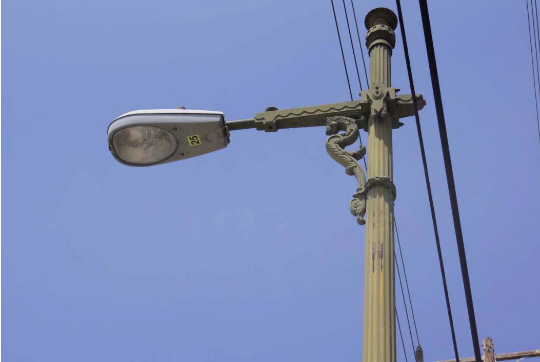
Figure 93. Olympic Boulevard Lamppost Detail, View West
