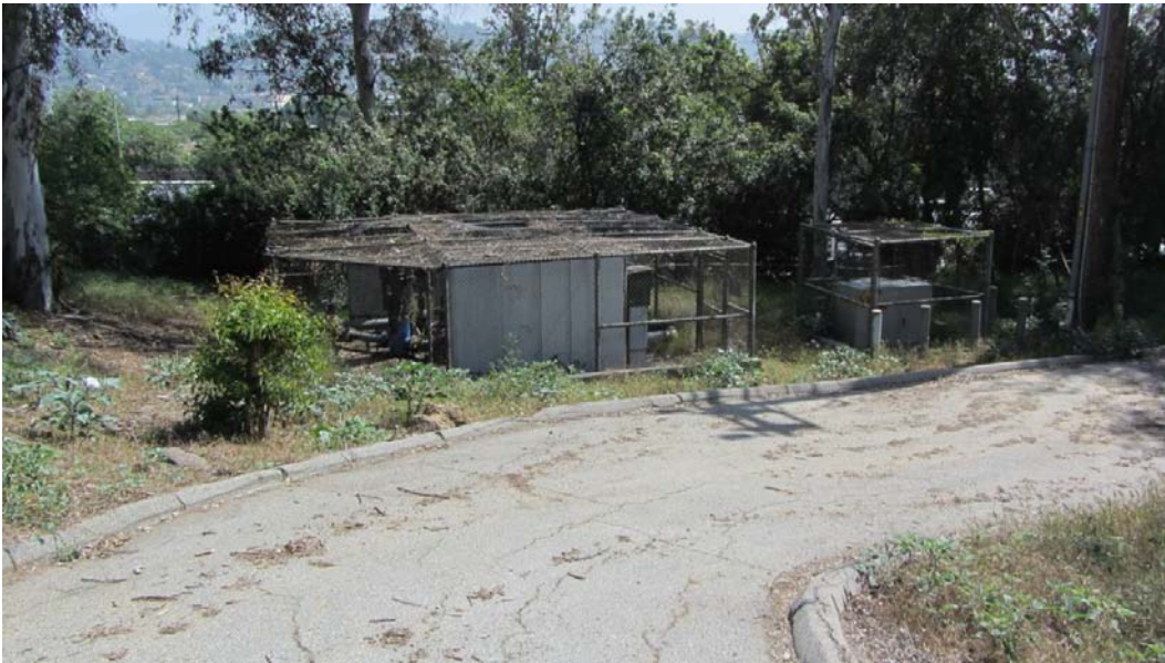
Figure 44. Existing Pumping Station at Proposed Location of New Recycled Water and Non-Potable Water Pumping Stations and Forebay Tank, View Northeast
