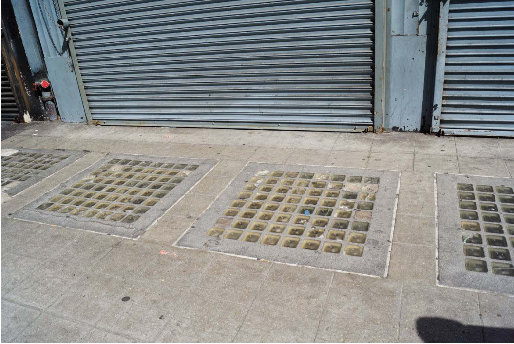
Figure 64. Vault Glass along Broadway between 8th and 9th Streets, View Southeast
