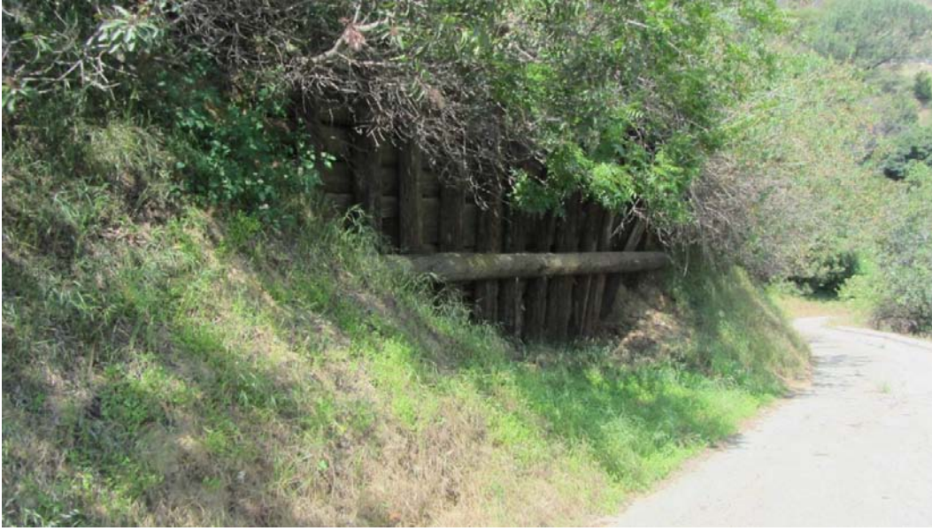
Figure 43. Wooden Retaining Wall, View toward Southwest
