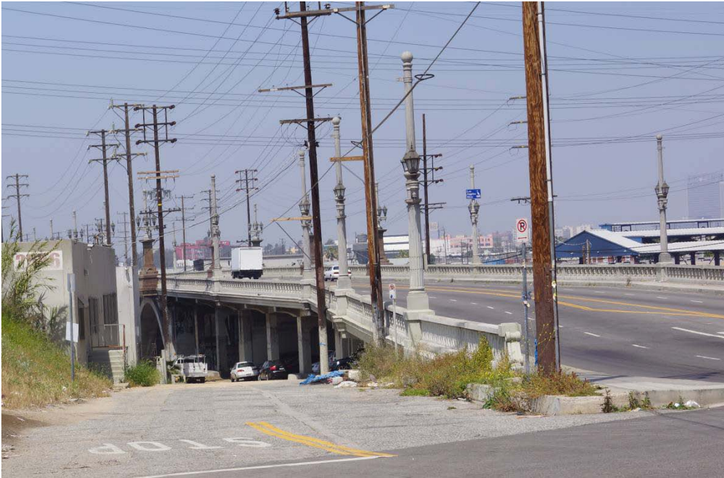
Figure 79. Olympic Boulevard Bridge/Viaduct, View West
