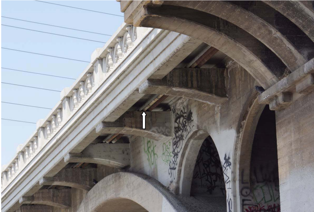
Figure 82. Olympic Boulevard Bridge, Existing Pipes, View Northwest
