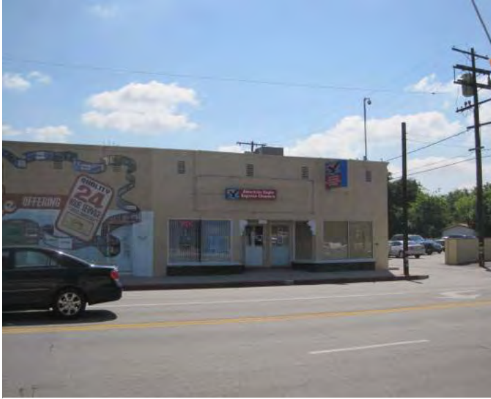
Whitsett Avenue and Magnolia Boulevard Southeast Plaza - American Eagle Cleaners
