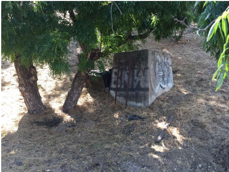
Figure 1. View north to Manhole Sewer structure (IMG_3632)
