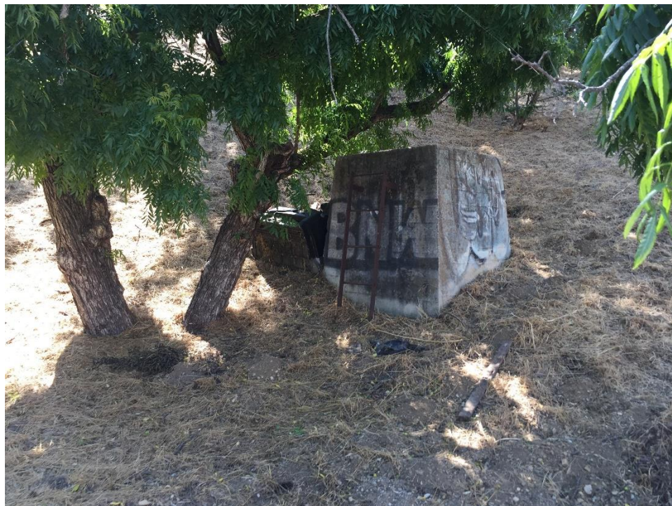
Figure 12. View north to Manhole Sewer structure (IMG_3632)
