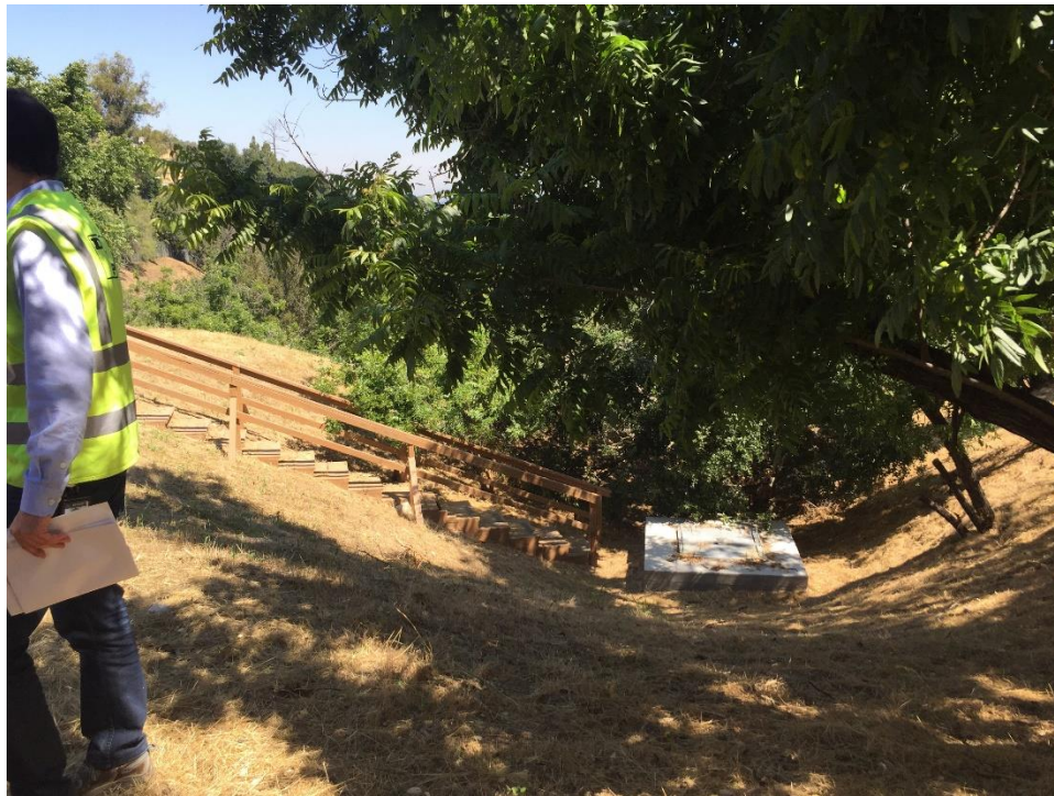
Figure 13. View east to Vault structure (IMG_3635)
