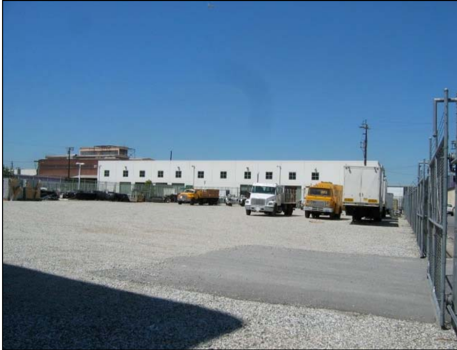
Figure 6: Project Overview: View towards west.
