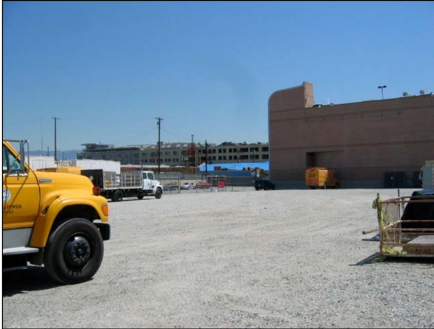
Figure 8: Project Overview: View towards northeast.
