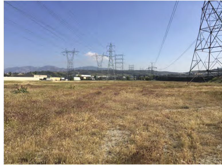
Center portion of the alignment, where the alignment crosses an industrial area in the City of Santa Clarita, just south of the Santa Clara River.
