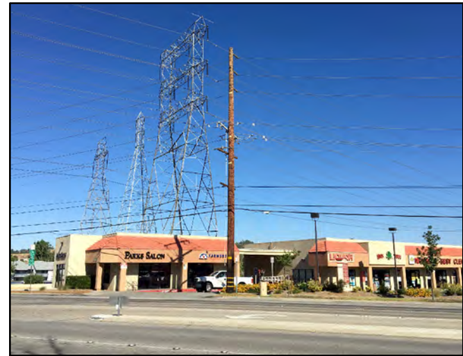
Photo J: View northwest from Bouquet Canyon Road to transmission lines and commercial development (Santa Clarita)
