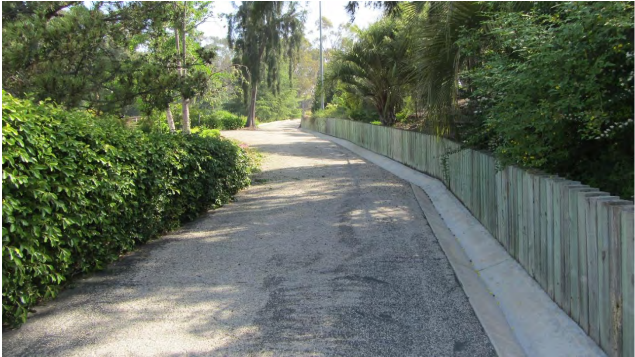
Figure 27. Utility Road Adjacent to Japanese gardens, View Northeast.
