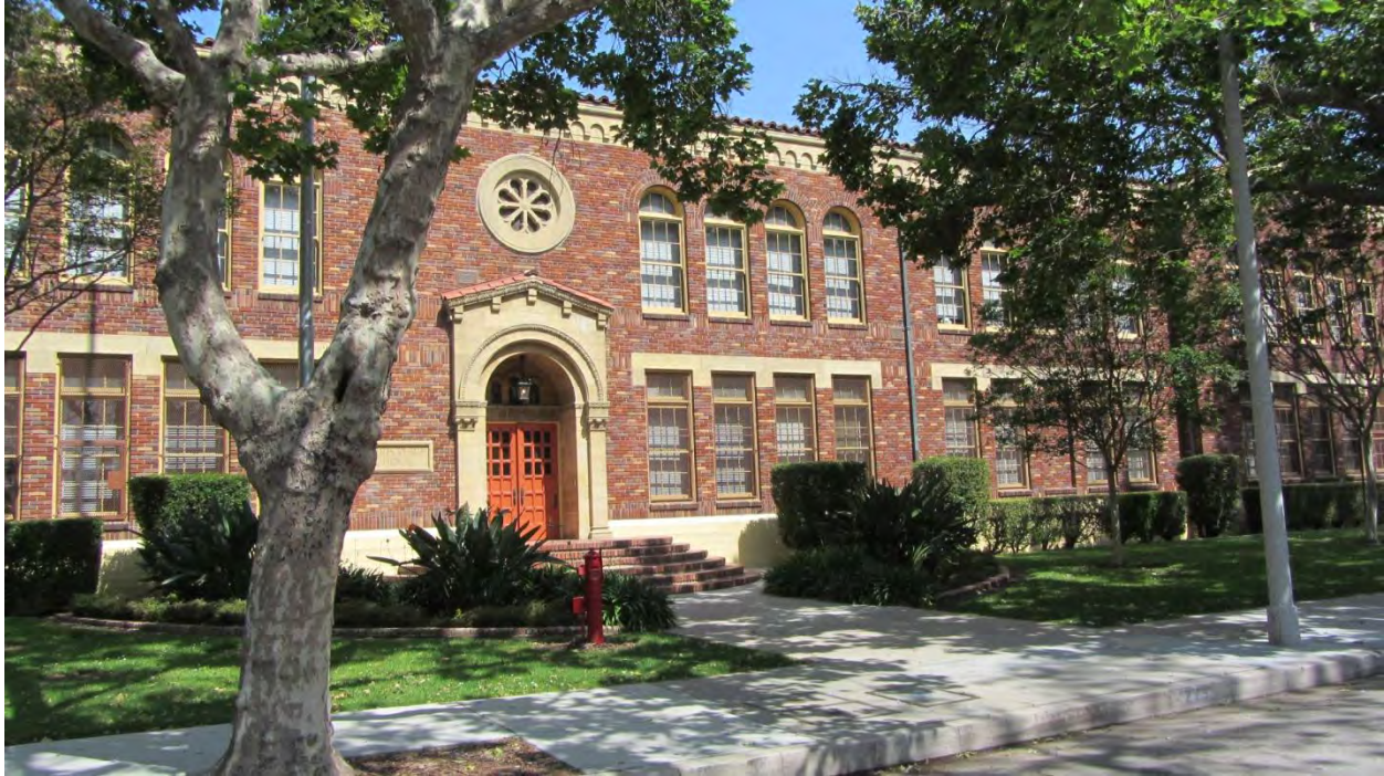
Figure 18. Dorris Place Elementary School, View Towards Northwest.
