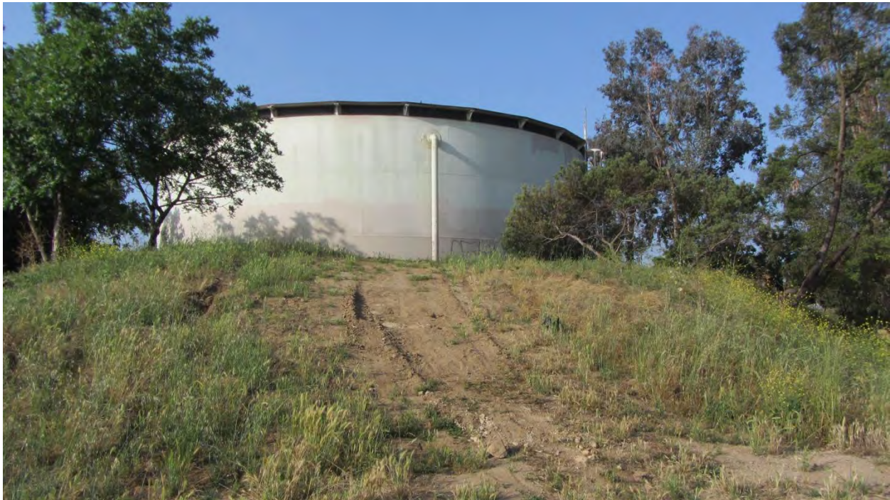
Figure 24. Existing Steel Water Tank, View Southwest.
