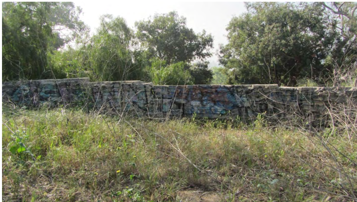
Figure 21. North Façade of Concrete Wall, View Southeast.
