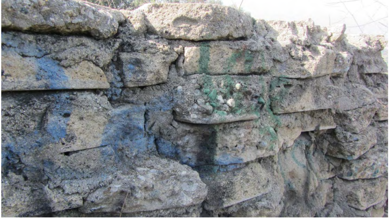
Figure 22. Close-up of Concrete Wall North Façade.
