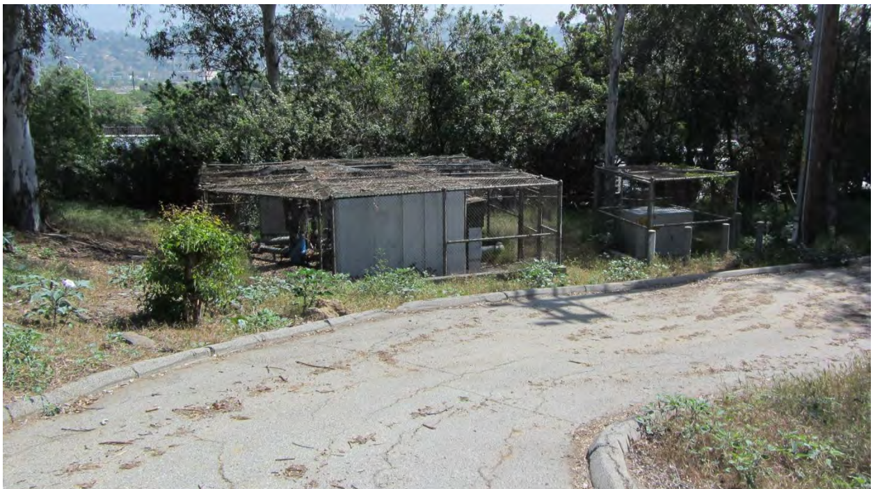
Figure 20. Existing Utility Structure at Proposed Location of Recycled Water Pumping Station, View Northeast.
