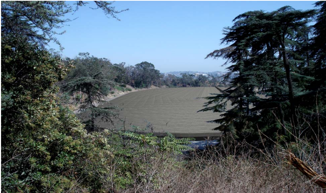
Figure 5-14 Proposed pedestrian view with Aluminum Cover from roadside on Grand View Drive
