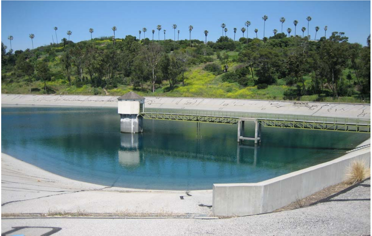
Figure 3.1-8 Photo 7: View of reservoir from southwest corner within the property
