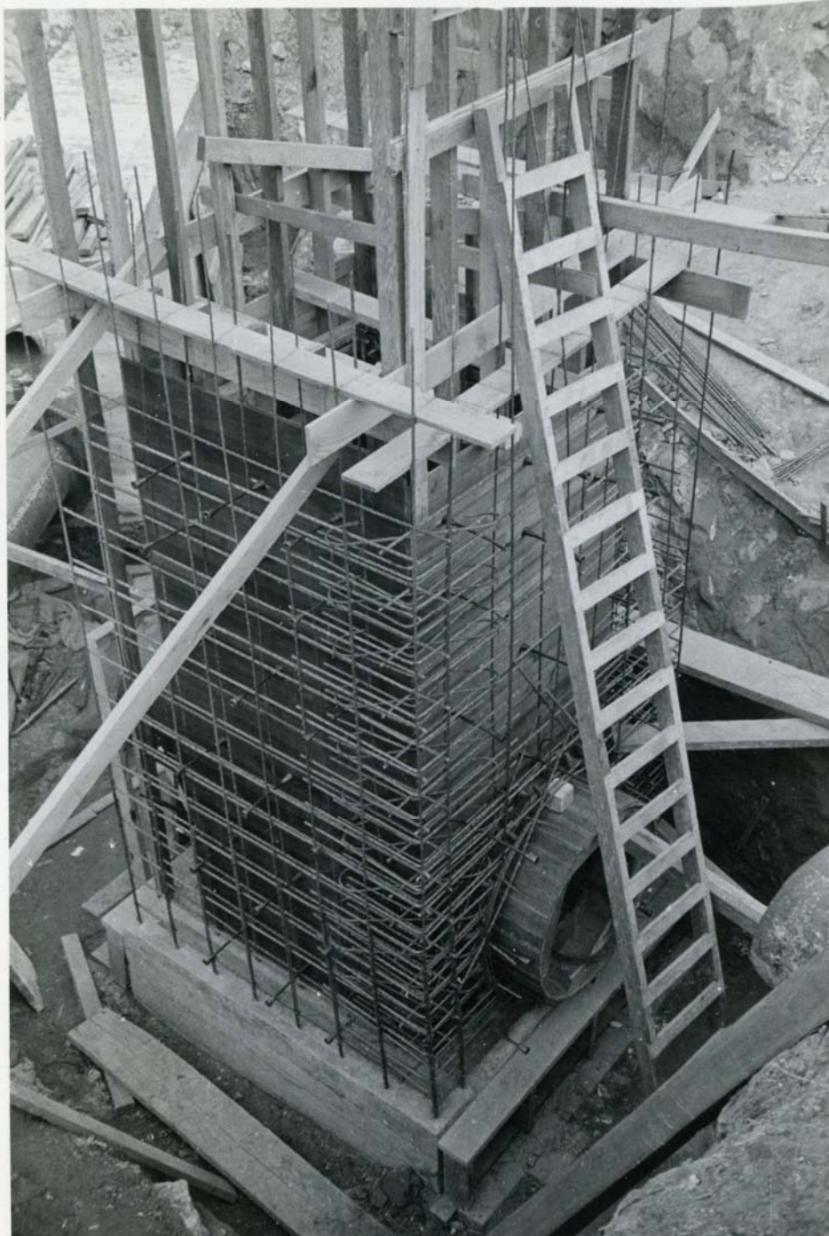
Plate 2. Inlet Tower Foundation January 10, 1942 (LADWP 1957:22)
