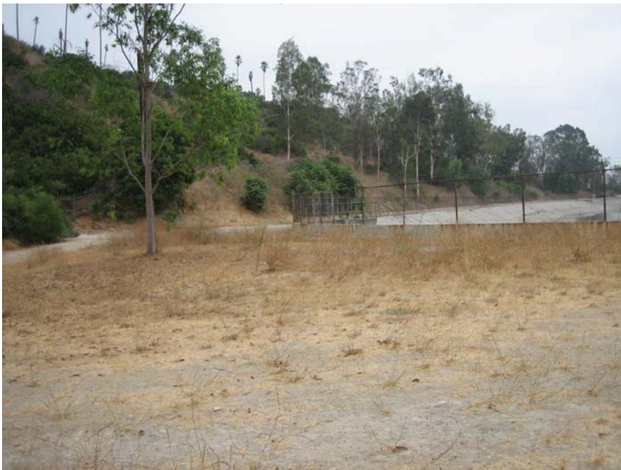
Plate 4. Pond/Staging Area at Northwestern End of Reservoir, View to East
