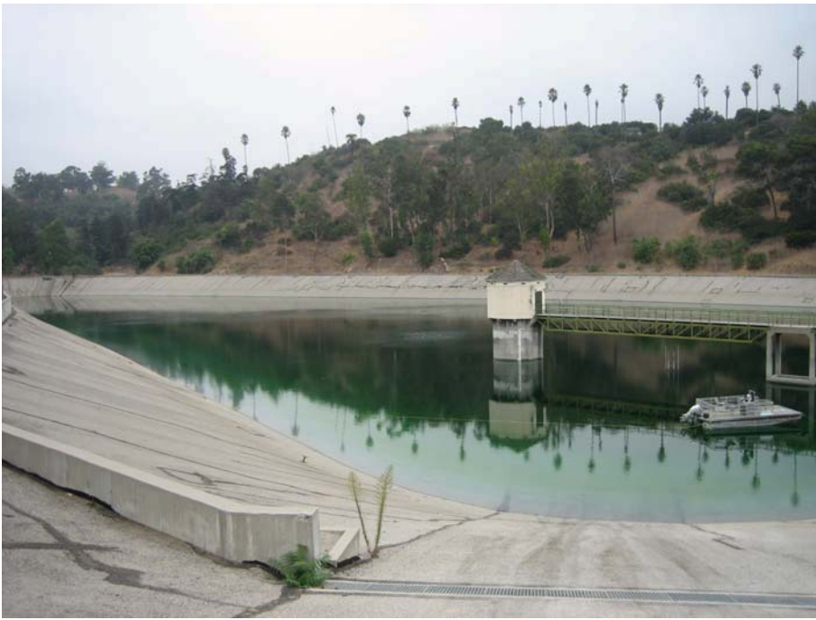
Plate 9. Overview of Reservoir, View to North
