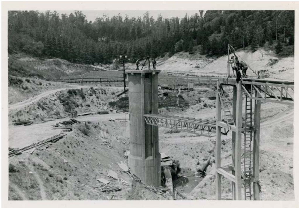
Plate 10. Outlet Tower and Bridge under Construction, May 13, 1942 (LADWP 1957:28)
