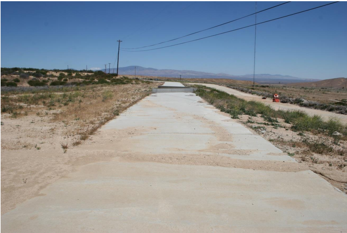
Plate 3. Overview of P-19-002105H, Los Angeles Aqueduct, Feature 1
