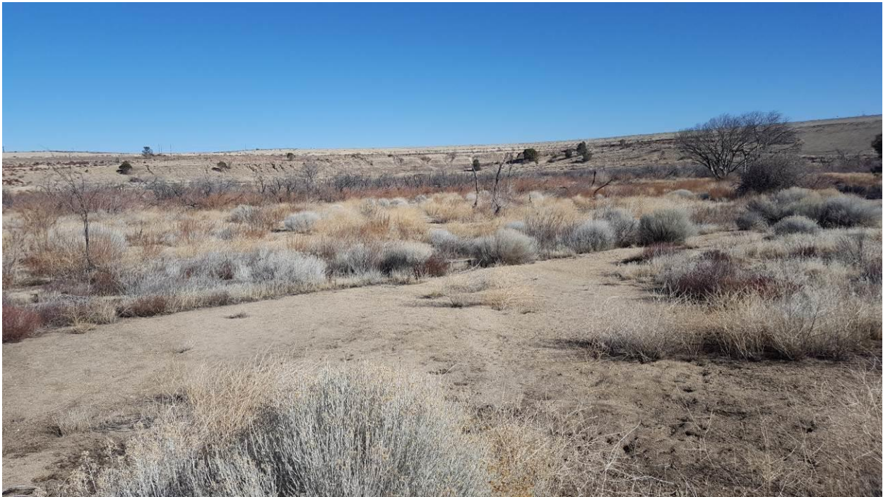
Photo 10: West-facing view across the bottom of dry Fairmont Reservoir #1, with the western bank of the reservoir visible in the background (photo taken January 17, 2017).
