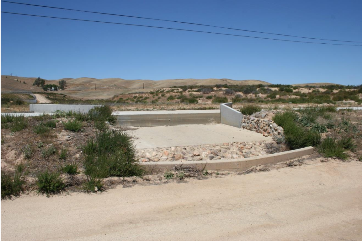
Plate 6. Overview of P-19-002105H, Feature 2, Los Angeles Aqueduct Spillway
