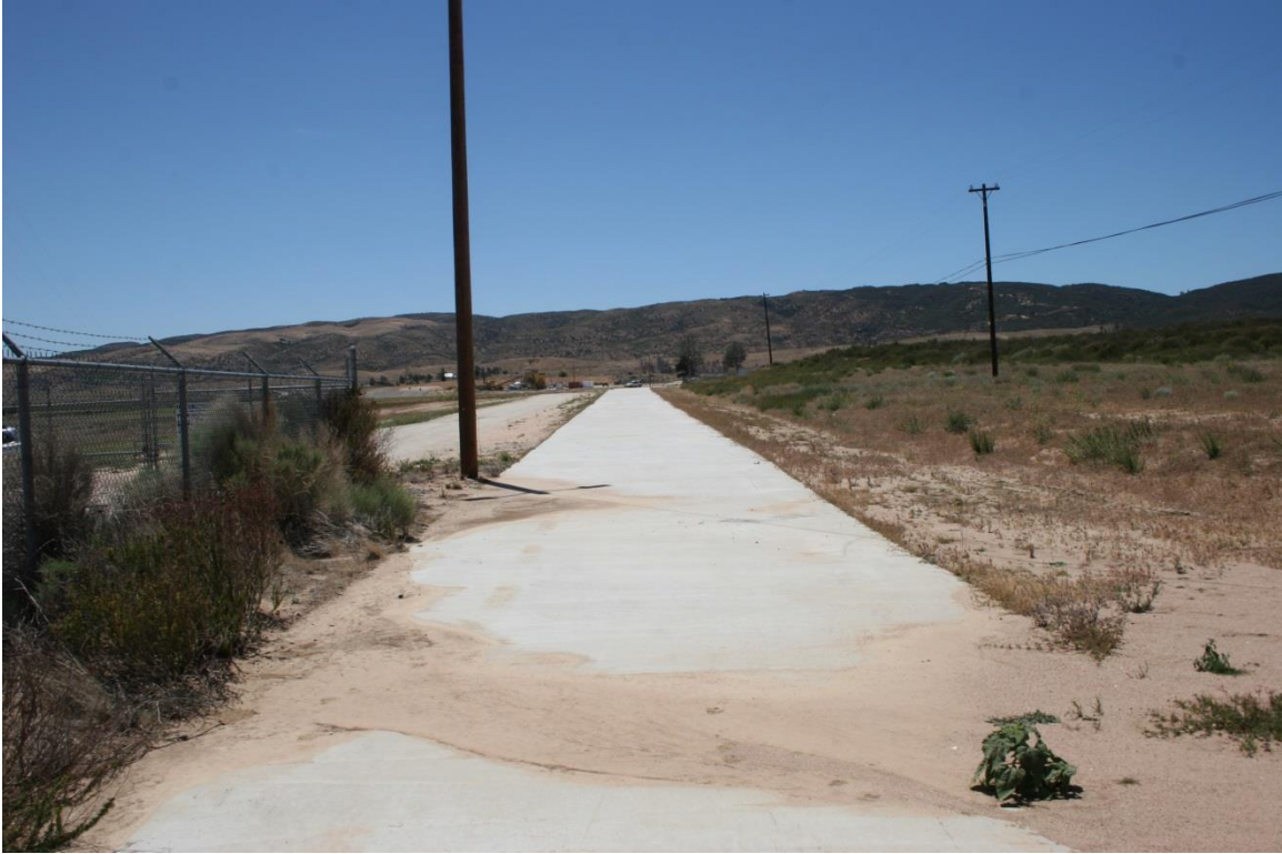
Plate 4. Overview of P-19-002105H, Los Angeles Aqueduct, Feature 1
