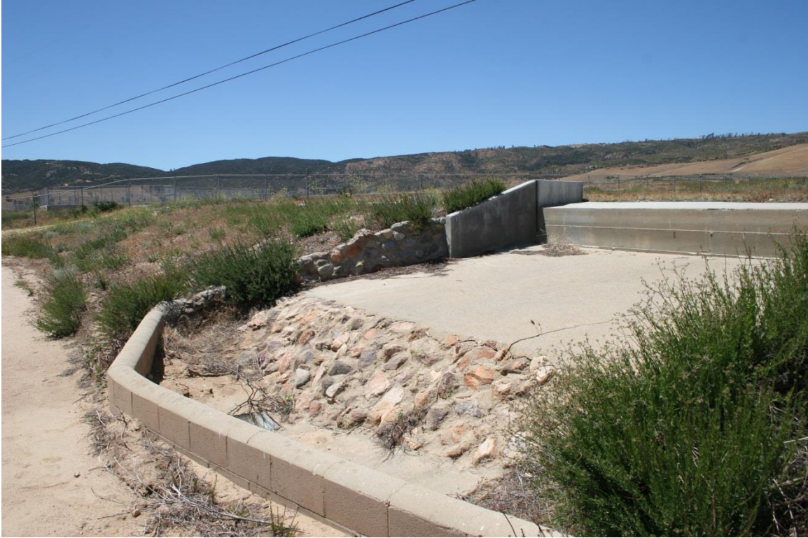
Plate 7. Overview of P-19-002105H, Feature 2, Los Angeles Aqueduct Spillway
