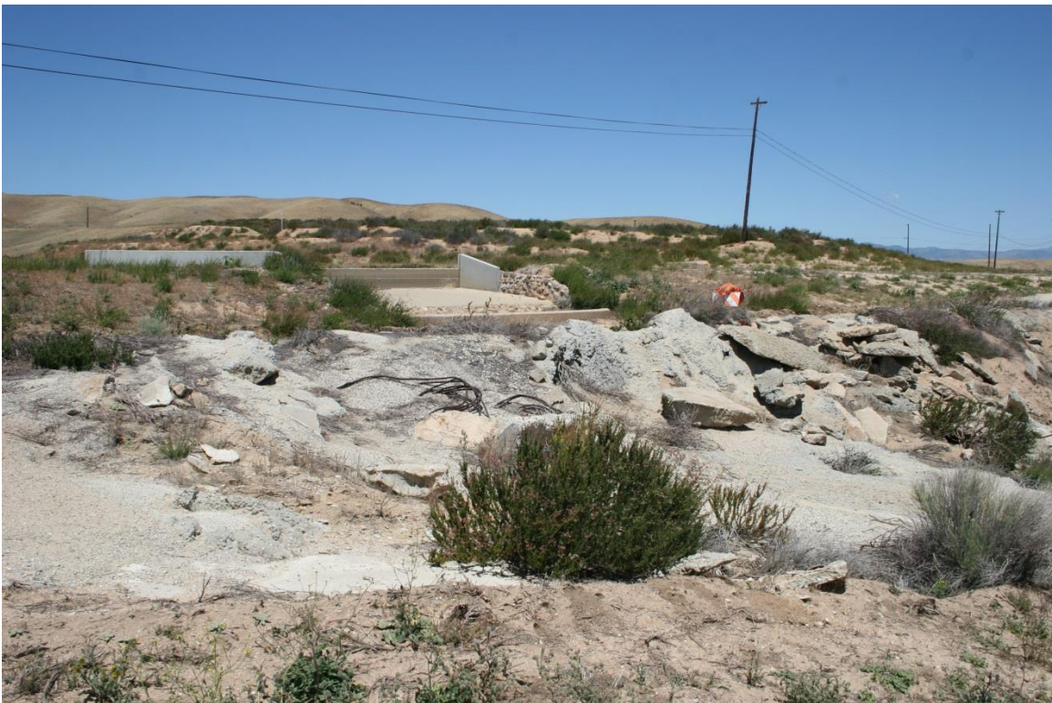
Plate 8. Overview of P-19-002105H, Feature 2, Los Angeles Aqueduct Spillway Drainage
