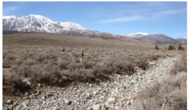
Unlined spillway, looking northwest
