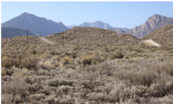
Grant Lake Dam (on left) and concrete spillway (on right), looking southwest from proposed staging area
