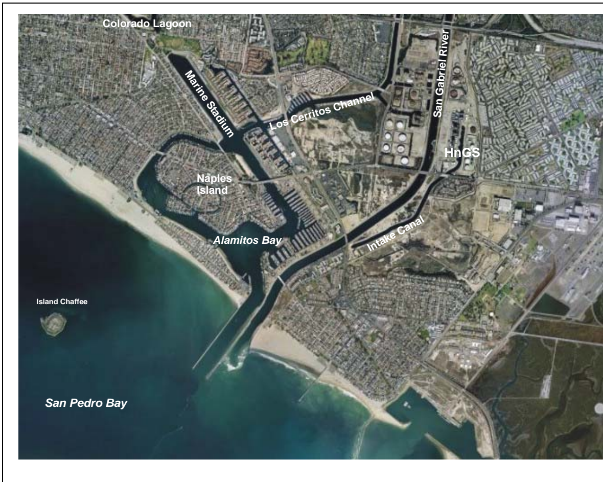
Figure 2.1-1. Aerial view of the HnGS and surrounding environment.
