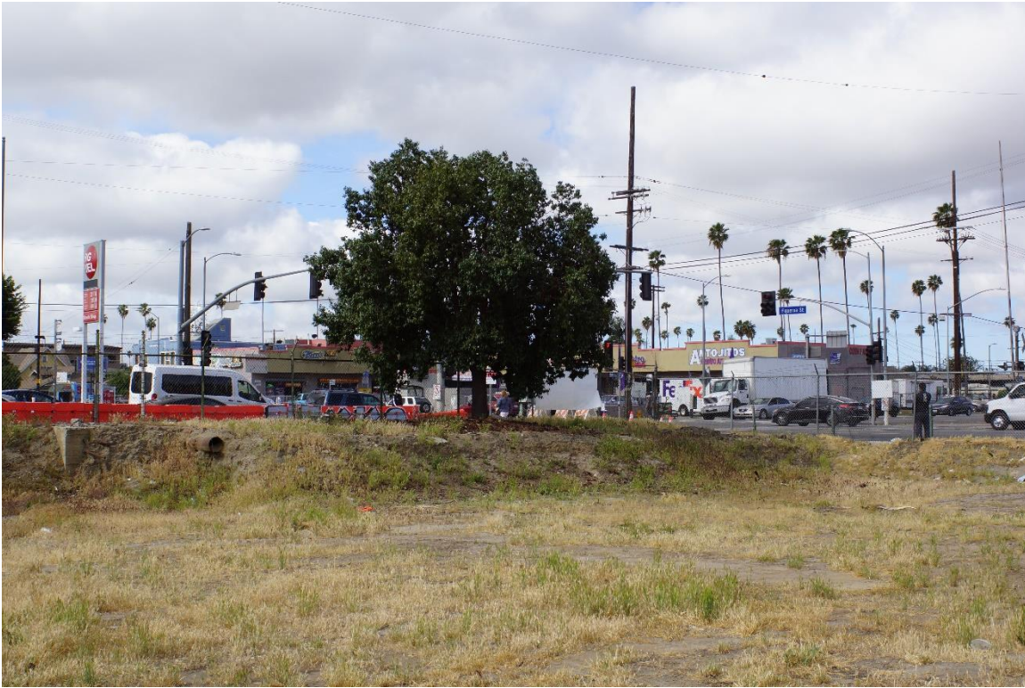
Plate 2: Building Foundation Location Overview, View Southwest
