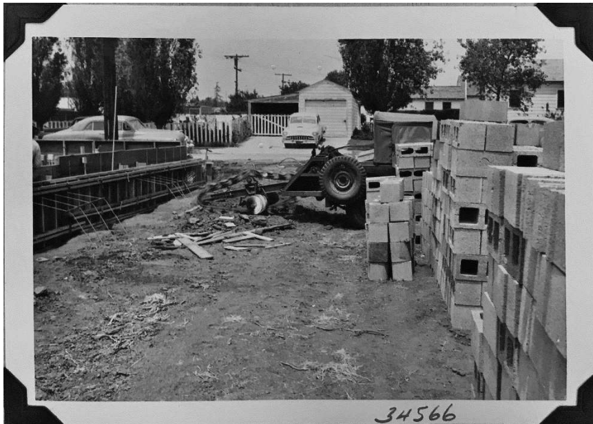
West Los Angeles Headquarters, Building 1, foundation; May 22, 1953 (LADWP No. 34566)
