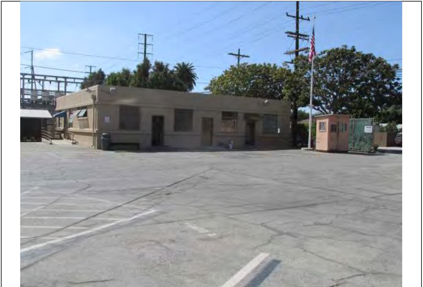
Figure 14. View of the northeast (main) and southeast elevations, looking west. 10/11/2017 (IMG 4050)
