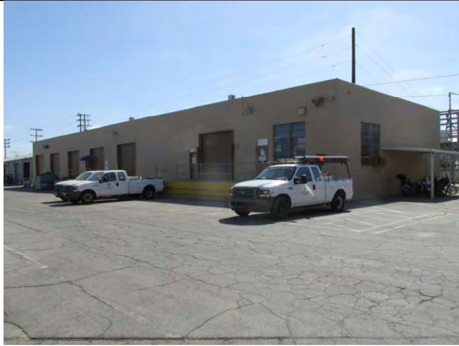
Figure 3. Building 2. View to south. 10/11/2017 (IMG 4077)
