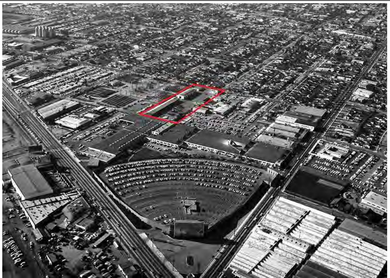
Figure 8. Bird's eye view of the Olympic Drive-In Theater with the Department of Water and Power headquarters highlighted, and the Receiving Station K and transformer yard to the left. Note that Building 5 had not yet been built. Photographer: Howard D. Kelly. January 15, 1962. (LAPL 00103040)
