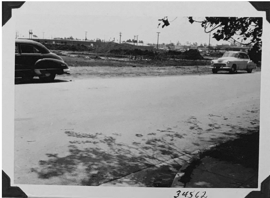
Clearing site at LADWP West Los Angeles Headquarters, May 8, 1953. (LADWP No. 34562)
