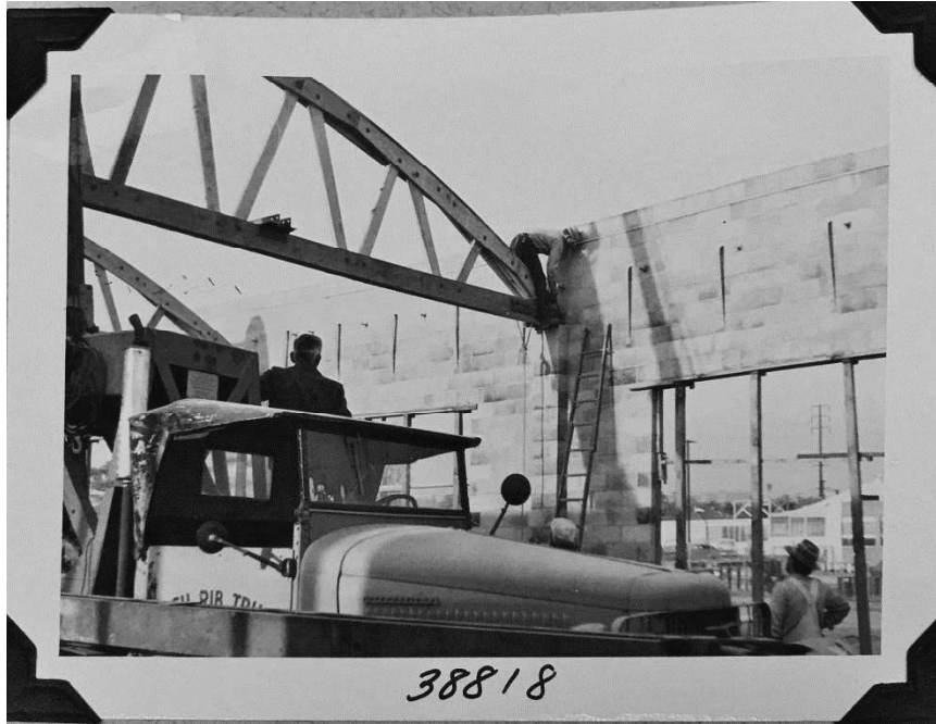
West Los Angeles Headquarters, Building 2 (warehouse), setting of roof truss – Arch Rib Truss Co; December 17, 1953 (LADWP No. 38818)
