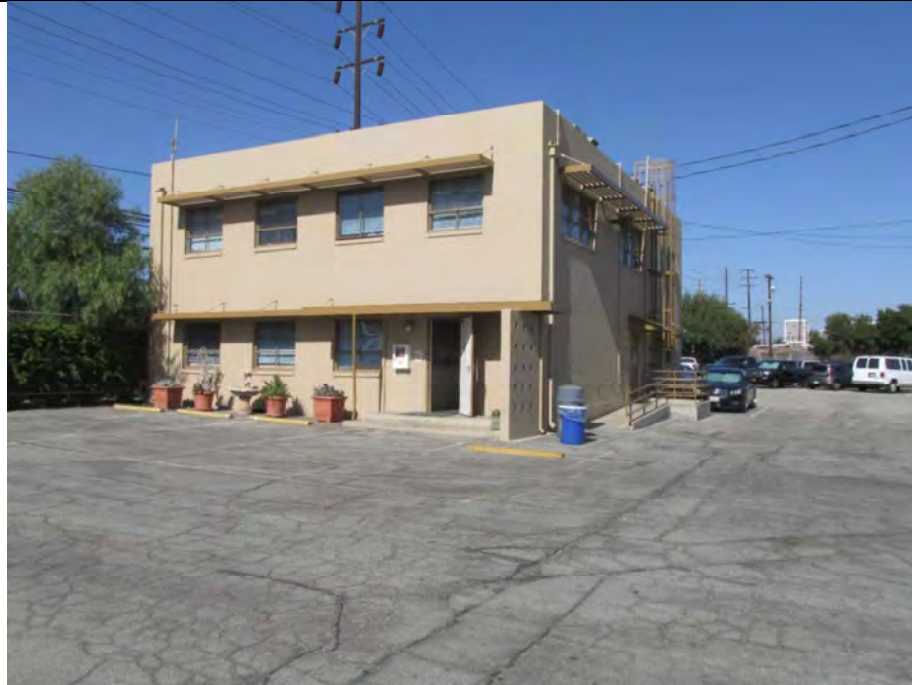
Figure 5. Overview of Building 4. View to North. 10/11/2017 (IMG 4138)
