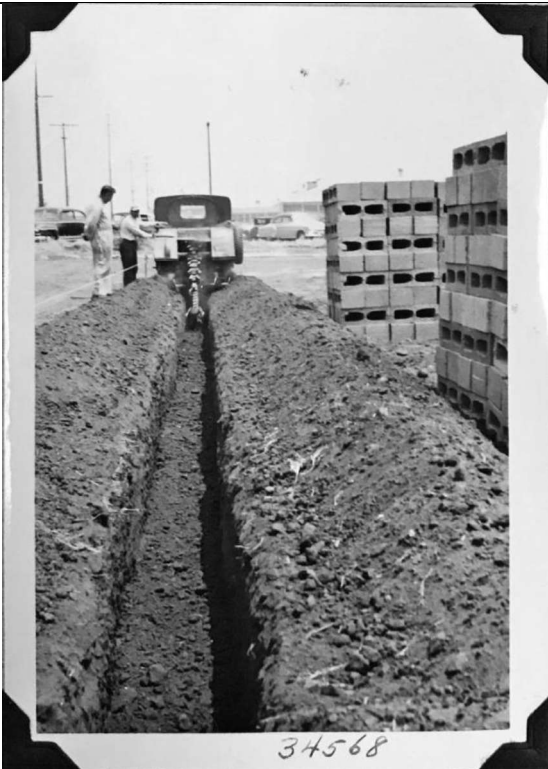
West Los Angeles Headquarters, Building 1, foundation; May 22, 1953 (LADWP No. 34566)
