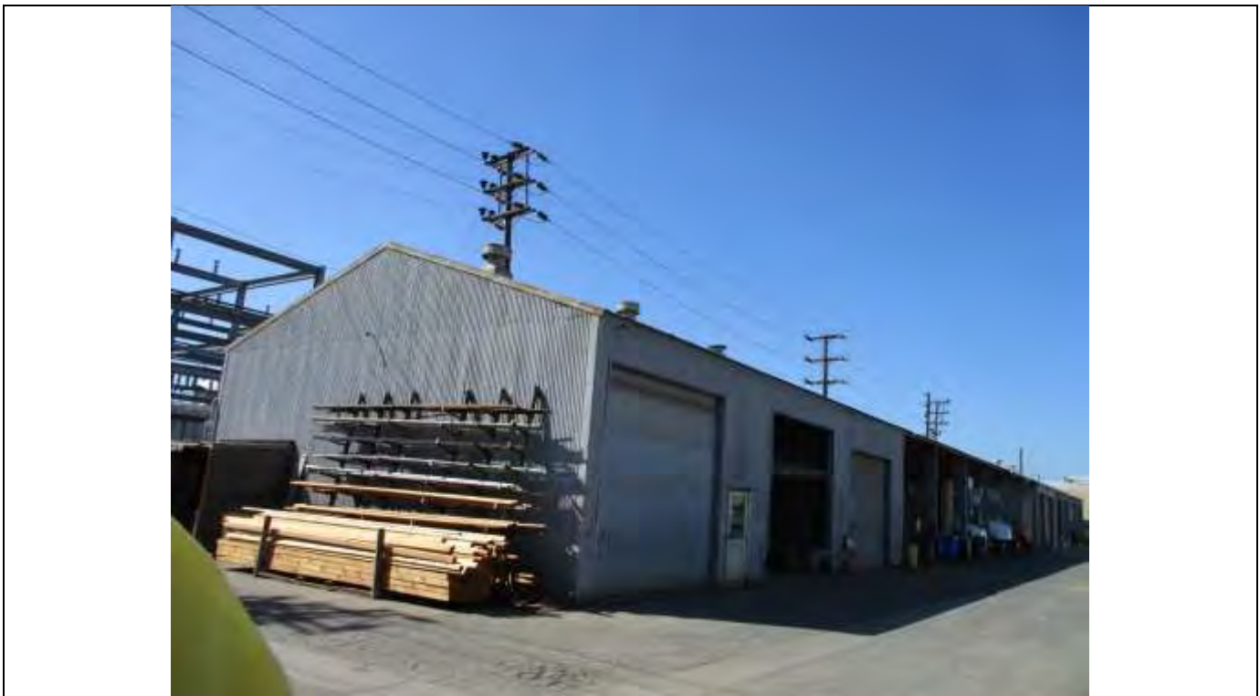
Figure 16. Building 3, view of the northeast (main) and southeast elevations, looking west. 10/11/2017 (IMG 0014)
