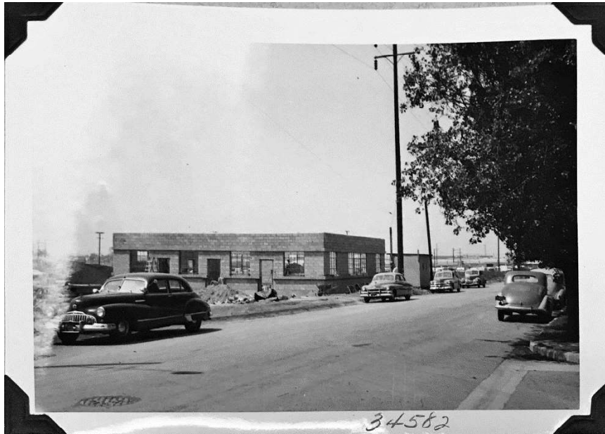
West Los Angeles Headquarters, Building 1, roofless; June 8, 1953 (LADWP No. 34576)
