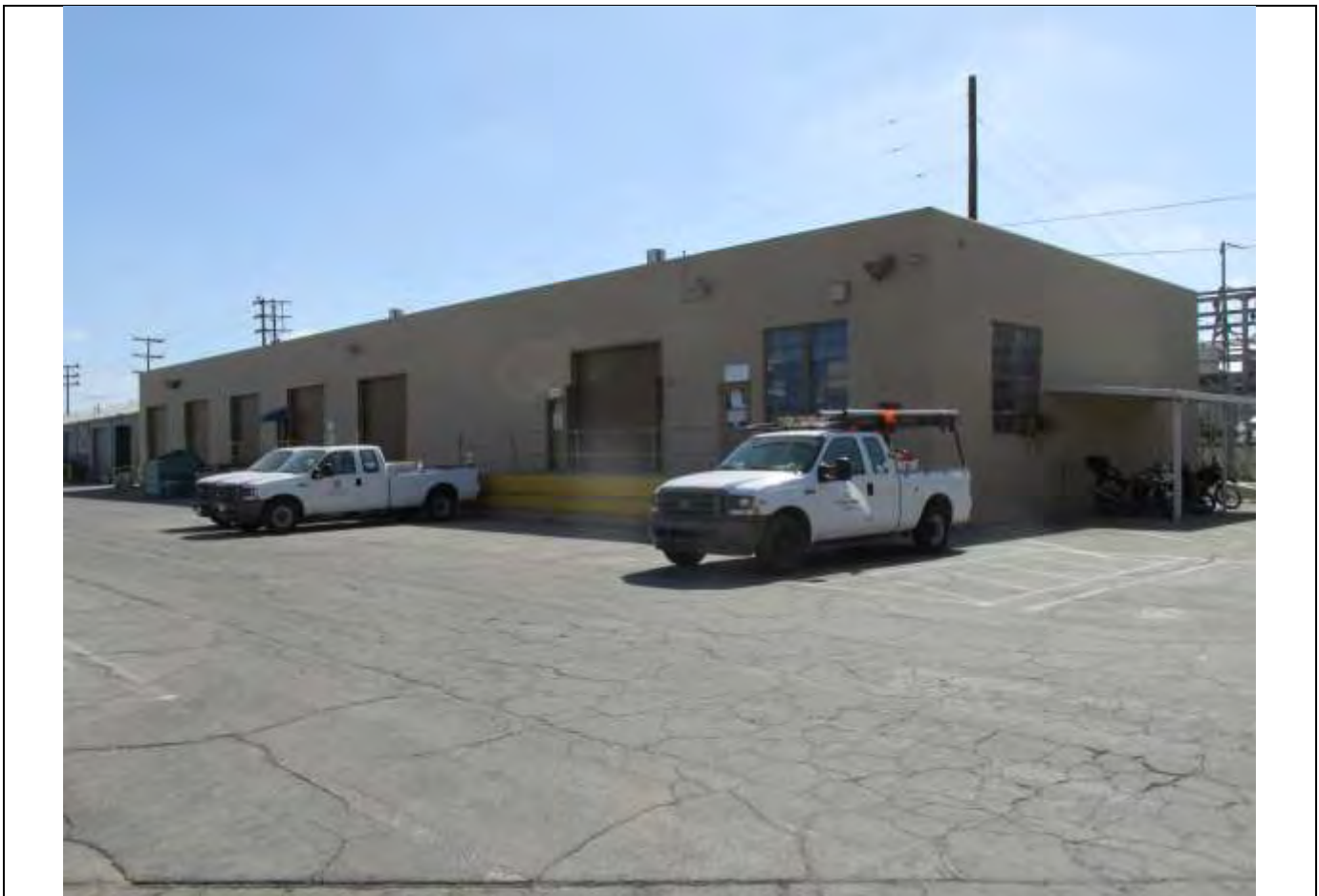
Figure 15. Building 2, view of the northeast (main) and northwest elevations, looking south. 10/11/2017 (IMG 4077)
