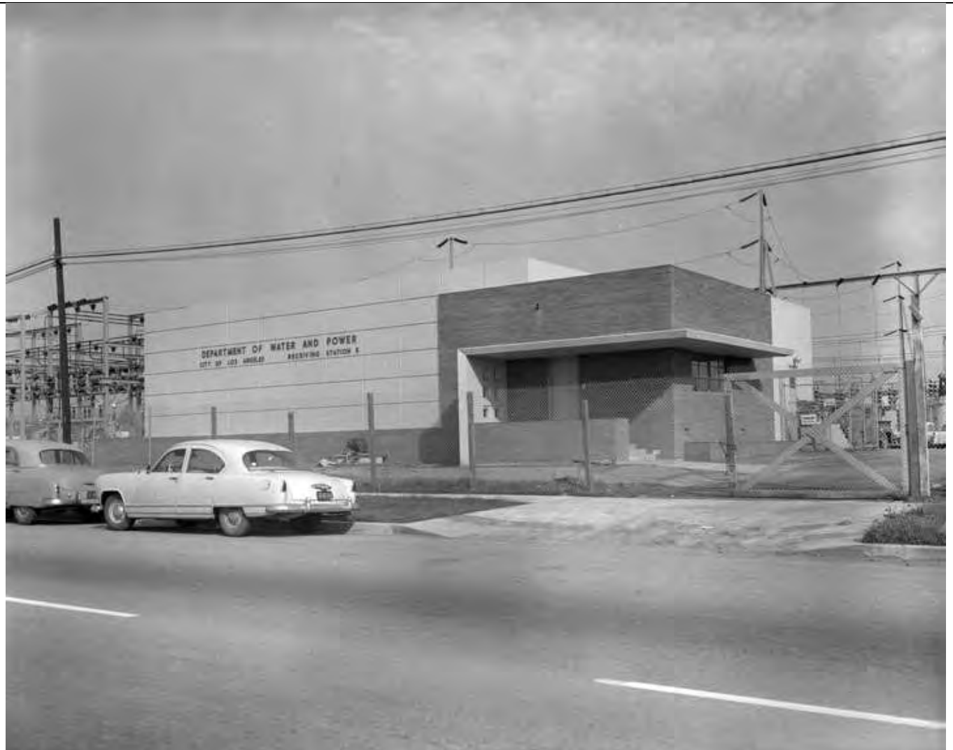
Figure 10. Receiving Station K at 1840 Centinela Avenue, built 1954, energized 1955. No date. (LAPL Barcode 1005633)
