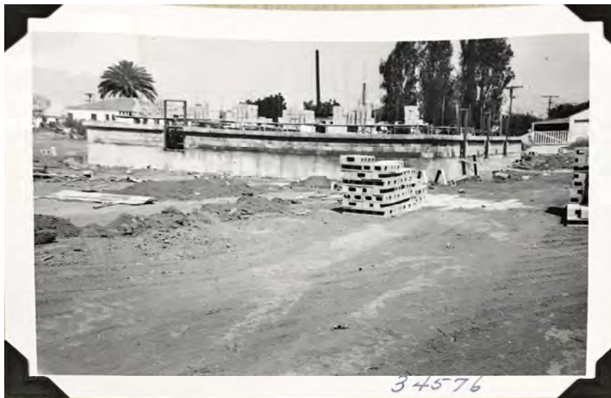
West Los Angeles Headquarters, Building 1, compacting backfill; June 1, 1953 (LADWP No. 34576)
