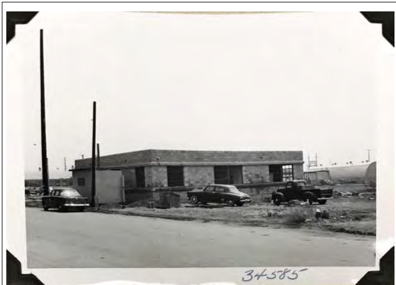
Figure 9. View to Building 1 (Locker Room) construction progress. July 23, 1953. (LADWP Record Center, Box WP24-24, File 13, Title “Underground Headquarters & Overhead Districts, 1953–1954 (Book 118)”, Photo Number 34585)
