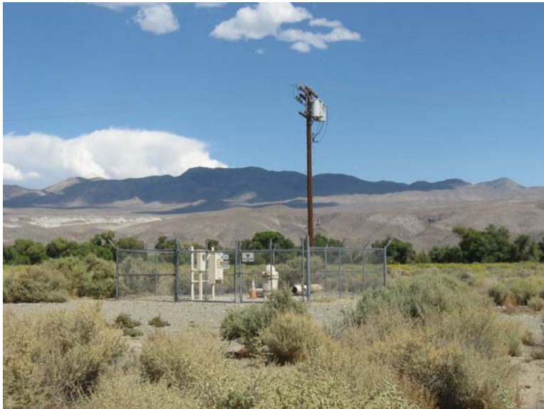
Figure 6 Existing Well W375 Conditions
