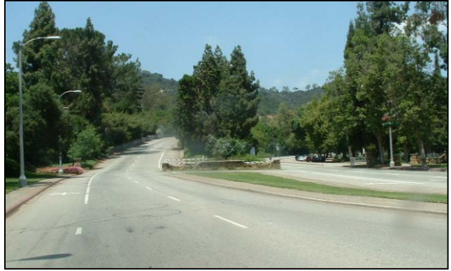
Photograph 31 - Looking north along the west side of Crystal Springs Drive from just north of Los Feliz Boulevard
