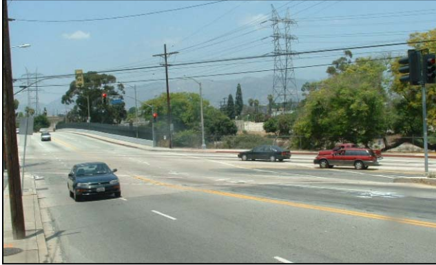
Photograph 39 - Looking northeast along the north side of Glendale Boulevard toward Riverside Drive
