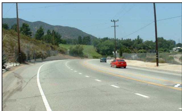
Photograph 5 - Looking west along the south side of Forest Lawn Drive from west of Zoo Drive
