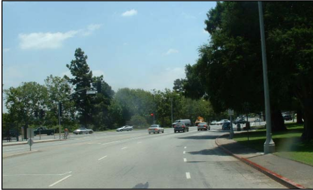
Photograph 32 - Looking south along the west side of Crystal Springs Drive toward Los Feliz Boulevard
