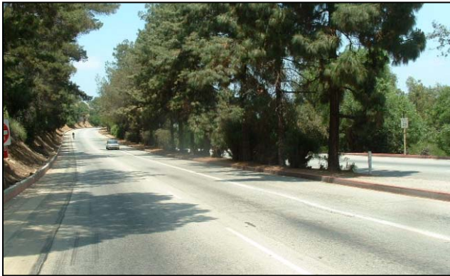
Photograph 28 - Looking north along the west side of Crystal Springs Drive south of Griffith Park Drive where Crystal Springs Drive becomes a four-lane divided roadway
