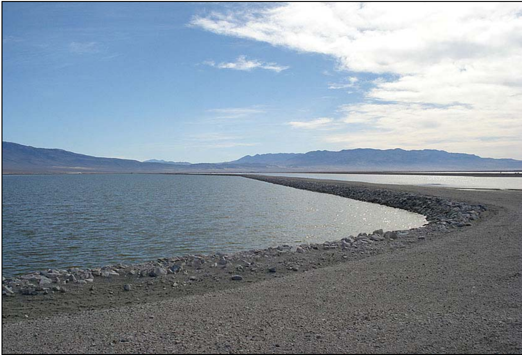
Ponded Shallow Flood — Looking southeast from southern edge of moat and row cell T32-1 towards adjacent ponds (cells T30-2, T29-1). (Photograph taken by EDAW on November 13, 2008)
