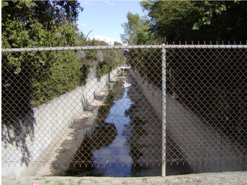
Pacoima Wash facing north from Parthenia Street east of Burnet Avenue
