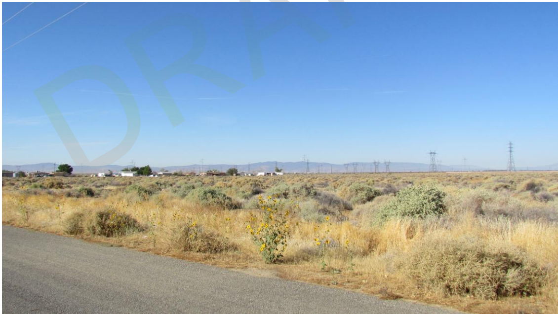
Photograph 2: Representative view of the Site and undeveloped property north of the Site, facing southwest from 100 th Street West. Residential structures (background) adjoin south of the Site.
