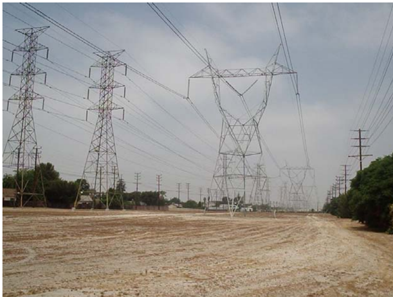
Figure 4-3 Whitnall Highway Utility Corridor
