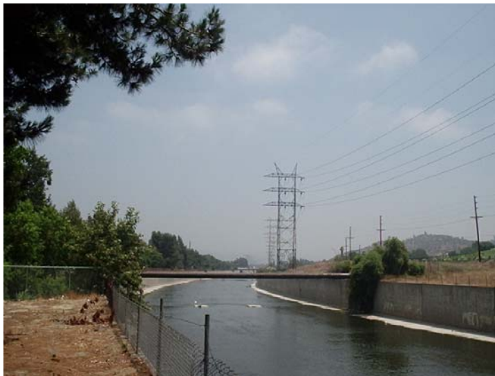
Figure 4-2 Existing Los Angeles River Pipe Bridge
