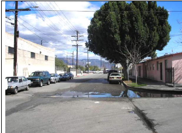
View to east on Hart Street, near Lankershim Blvd.
