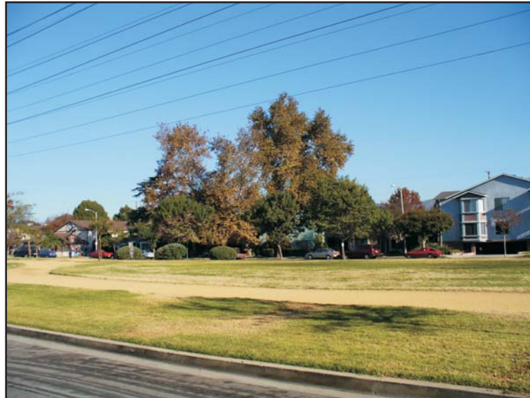
5. Transmission corridor on Kenwood Street
