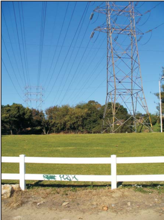
13. View northwest through corridor over Buena Vista Park
