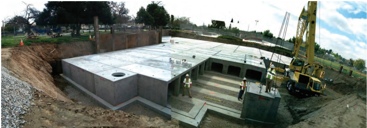
Garvanza Park Best Management Practices Project Infiltration Galleries
