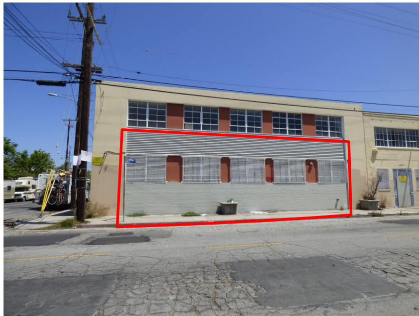
Figure 23 The south (side) elevation of Building C, view facing north, siding shown in red is an alteration
