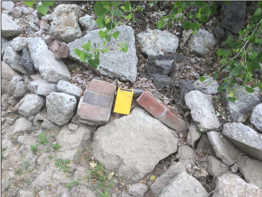
Figure 3. Close-up of asphalt and bricks lining east bank of drainage, Upper Northeast Drainage.
