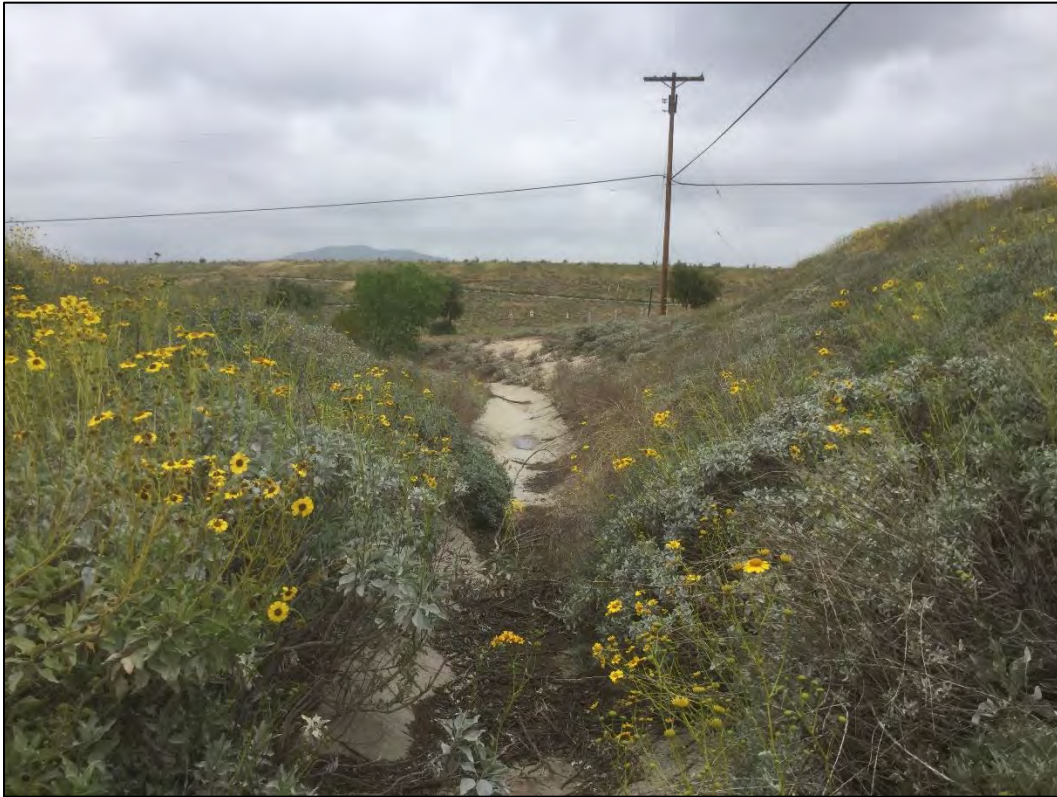
Figure 6. Overview of the Project Area, northeast terminus of drainage, LAR UV Plant Drainage
