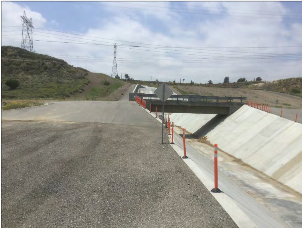
Figure 5. Developed concrete and asphalt ditch in middle Segment Bull Creek Extension.
