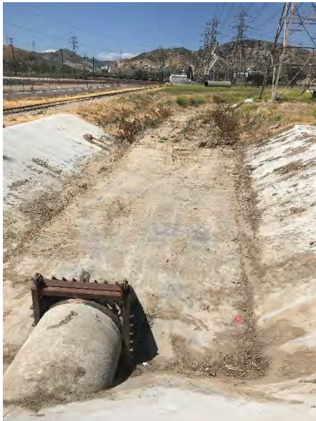
Photo 3: San Fernando Gate Drainage Feature
