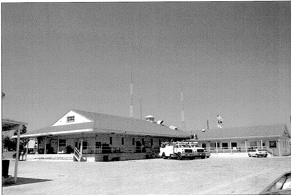
Rear West Side of Building 1 (view northwest)
