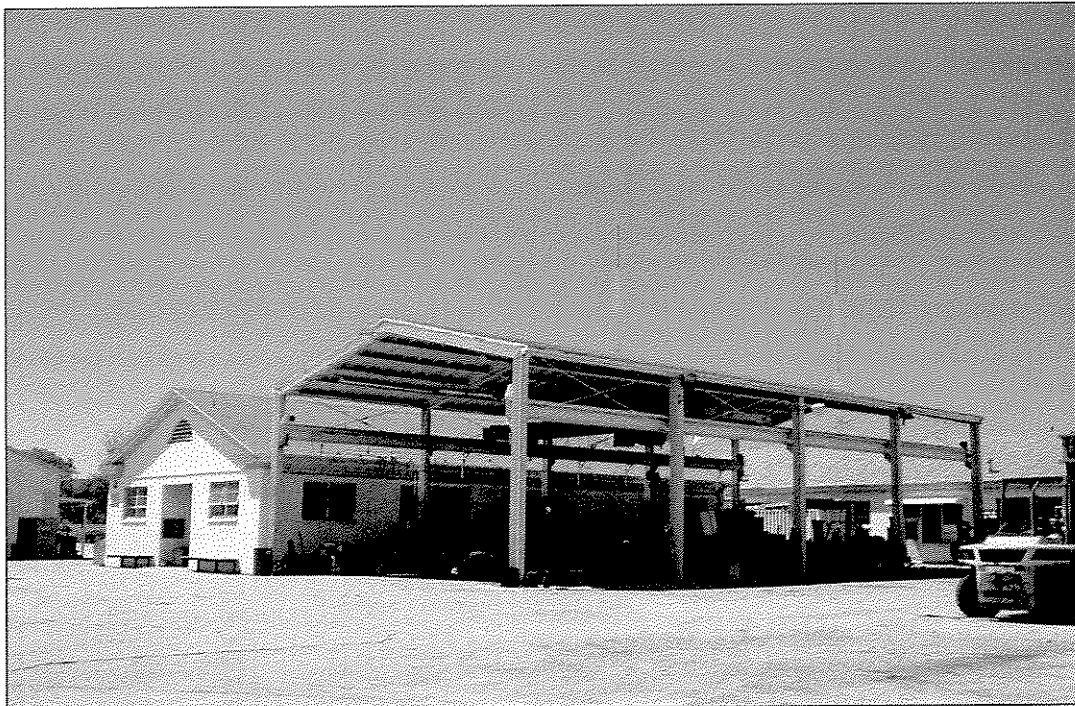
Building 6, Adjacent to Building 3 (view west)
