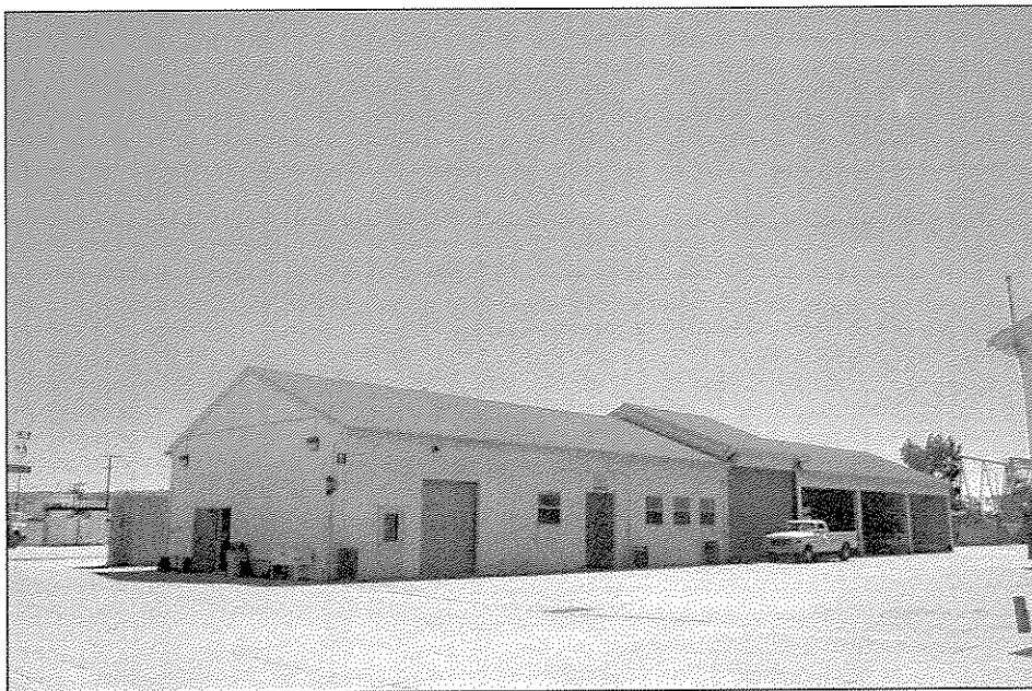
Front and East Side of Building 5 (view southwest)
